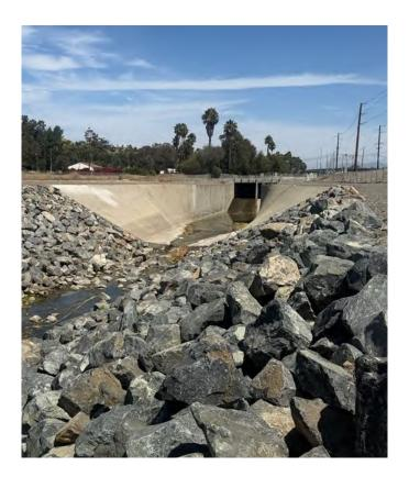
Figure 4  $\mid$  Rip Rap Lined Open Channel at Existing RCB Outfall
