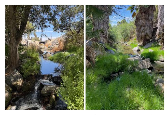
Figure 6 | Stable Vegetated Open Channel with Rip Rap Downstream of Culvert Outfall
