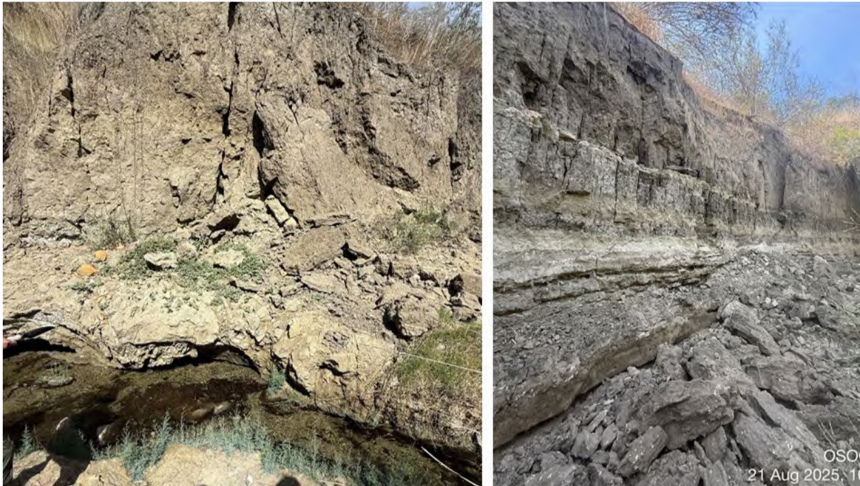
Figure 11 | Undercutting and Bank Collapse of Clay Soils
