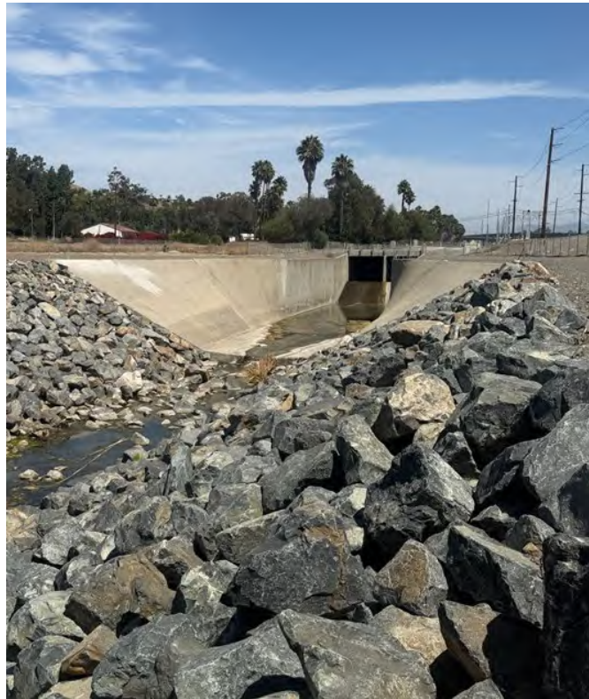
Figure 4 | Rip Rap Lined Open Channel at Existing RCB Outfall
