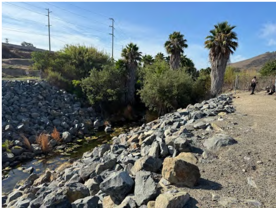
Figure 5 | Rip Rap Channel Transitions to Vegetated Channel with Rip Rap
