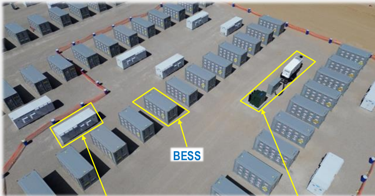
Power Conversion System (PCS) (Inverter & Transformer)
