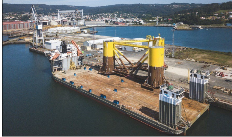
2) Loadout onto semi sub
