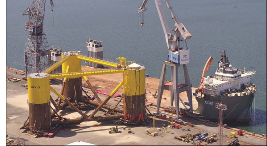
Example of a floating platform
