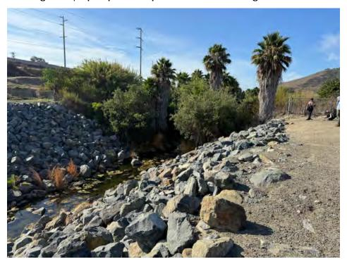
Figure 5 | Rip Rap Channel Transitions to Vegetated Channel with Rip Rap
