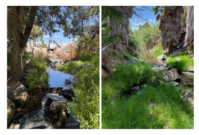
Figure 6 | Stable Vegetated Open Channel with Rip Rap Downstream of Culvert Outfall
