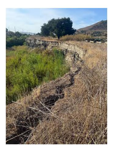
Figure 8 | Surface Cracks Along Channel Banks
