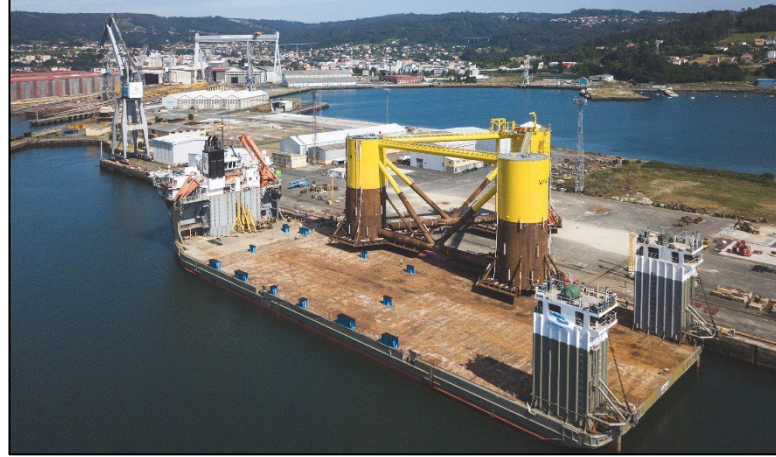
2) Loadout onto semi sub
