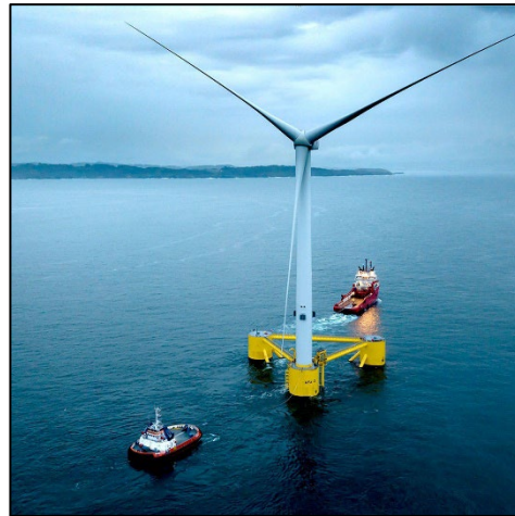
5) Tow to Installation Site
