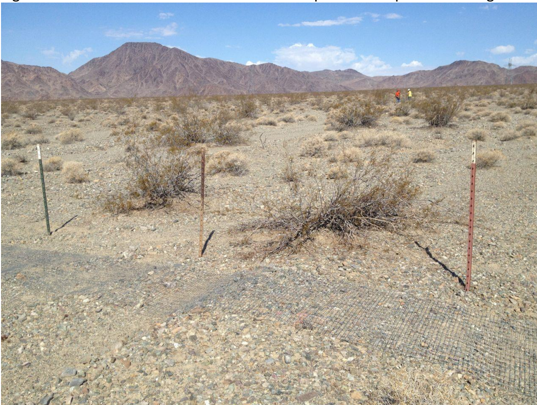
Figure 4. Well site and construction of tortoise-proof fence prior to drilling.
