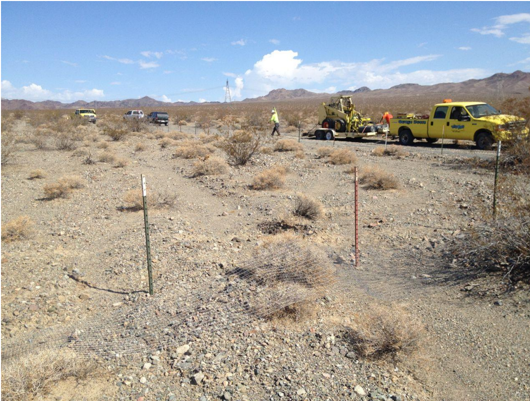
Figure 3. Well site and construction of tortoise-proof fence prior to drilling.
