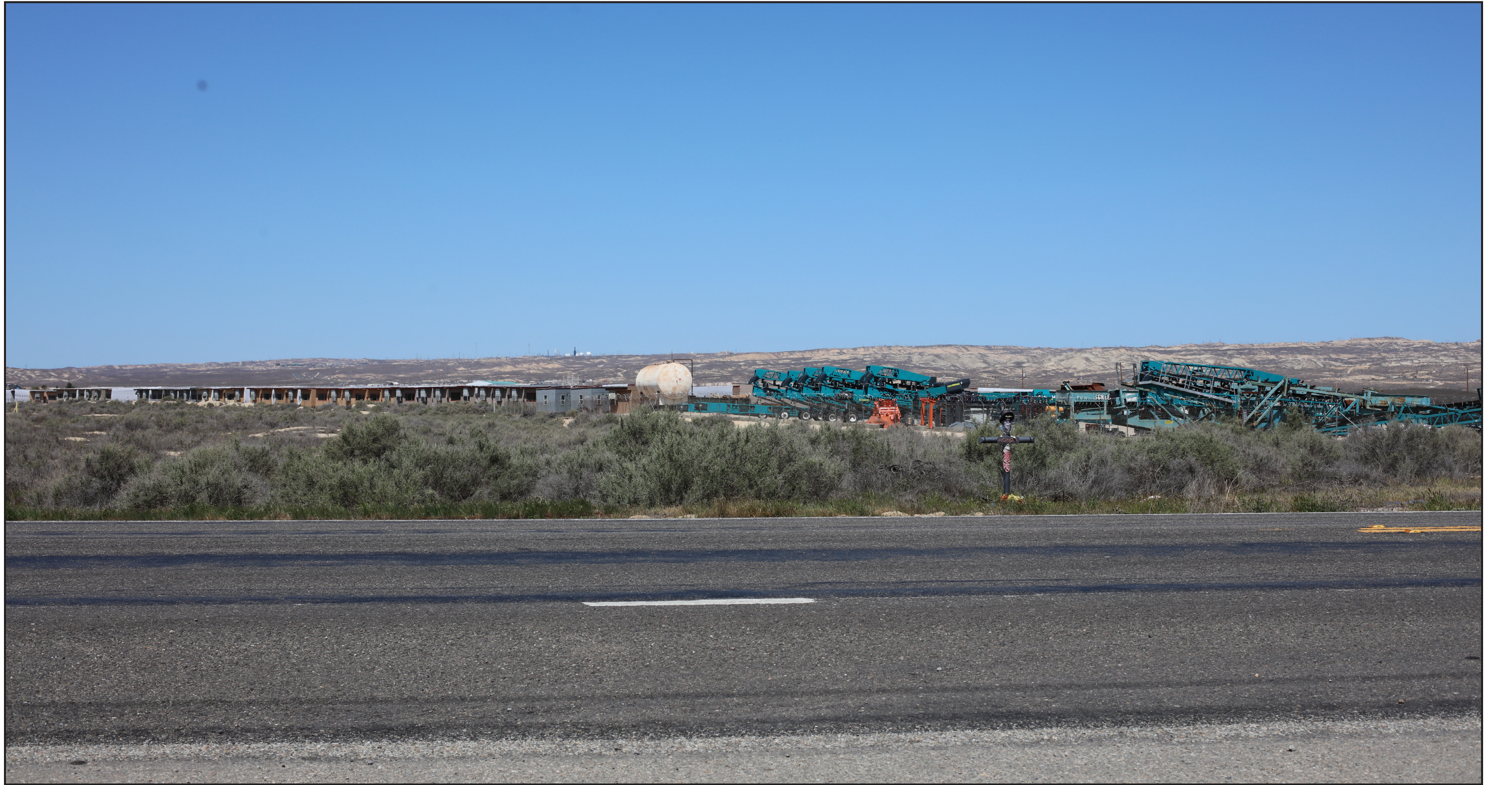
Existing Northwest View from California State Route 119.
