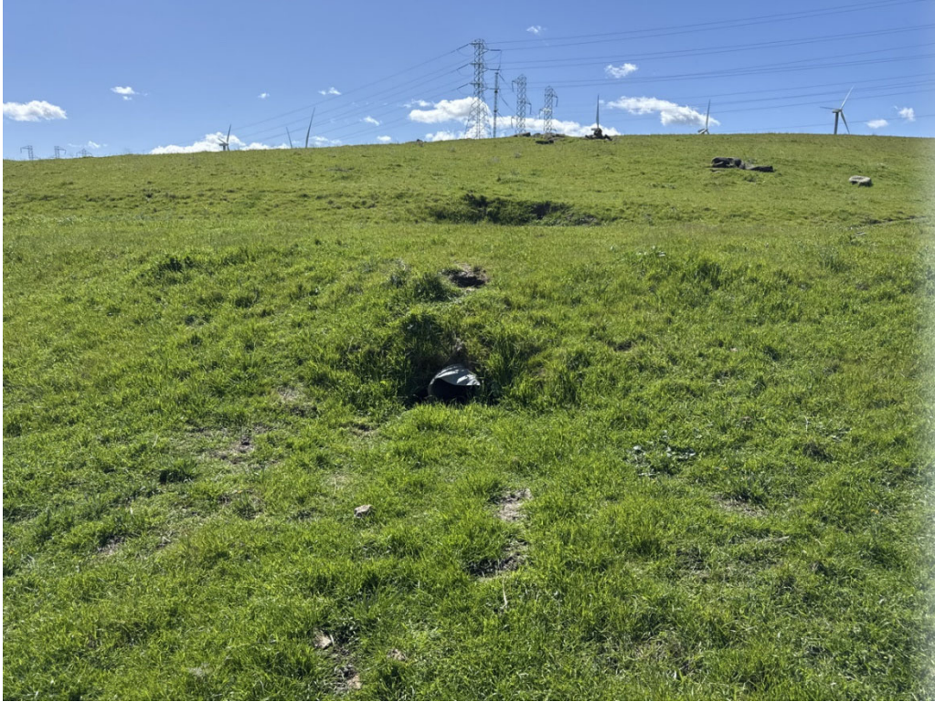
Photo 13: No aquatic resources observed at culvert outlet; facing south. Photo taken on March 18, 2025.
