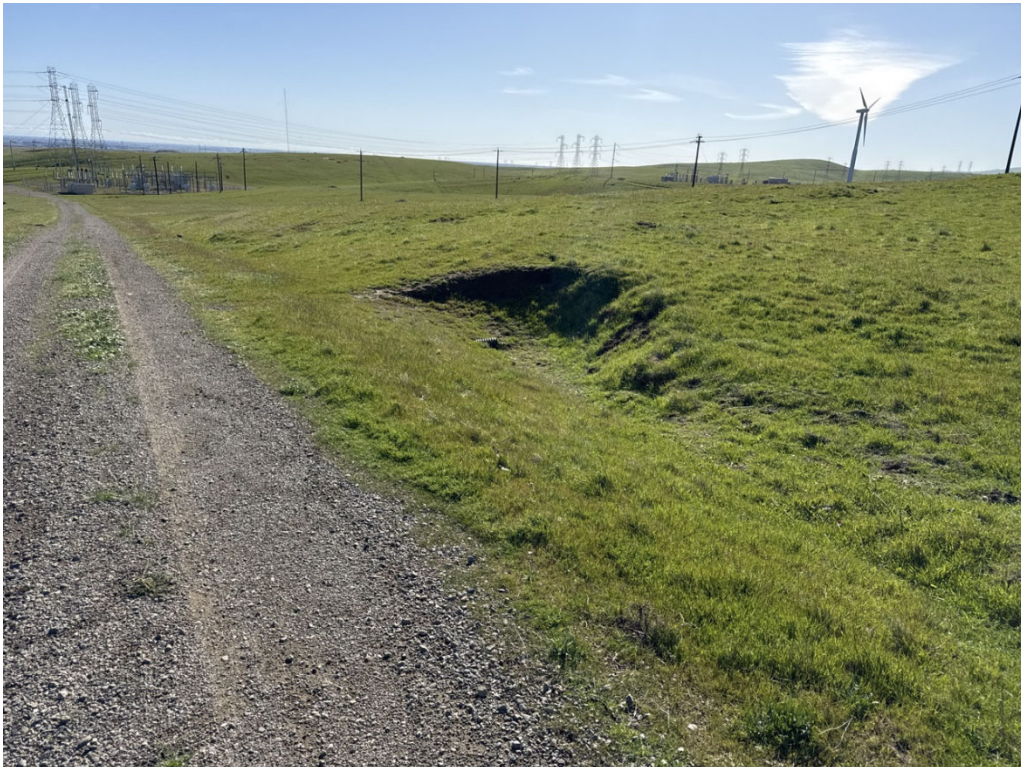
Photo 4: Culvert inlet along the south side of the existing access road. No aquatic resources were delineated in this area. Photo taken on March 18, 2025, facing east.
