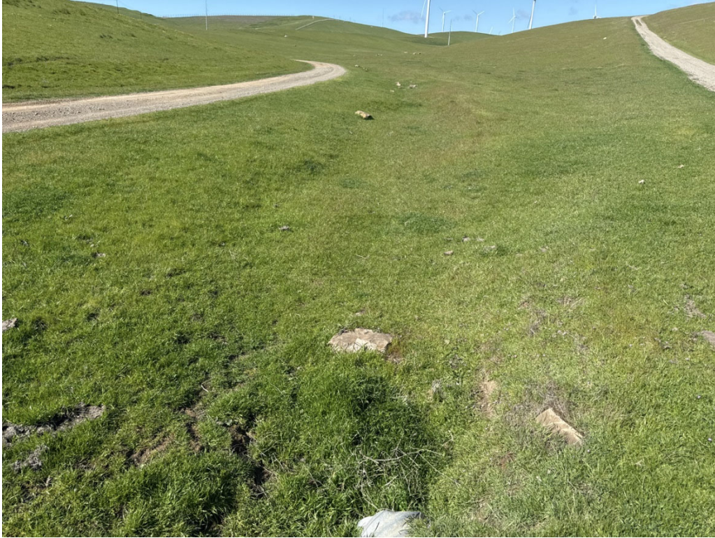
Photo 7: A vegetated swale at culvert outlet. No OHWM indicators or wetland indicators observed. Photo taken on March 18, 2025, facing southwest.
