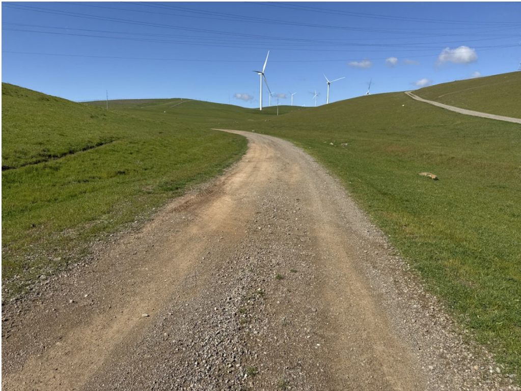
Photo 8: Photo taken at a mapped NHD flowline at the access road. No OHWM indicators observed. Photo taken on March 18, 2025, facing west.
