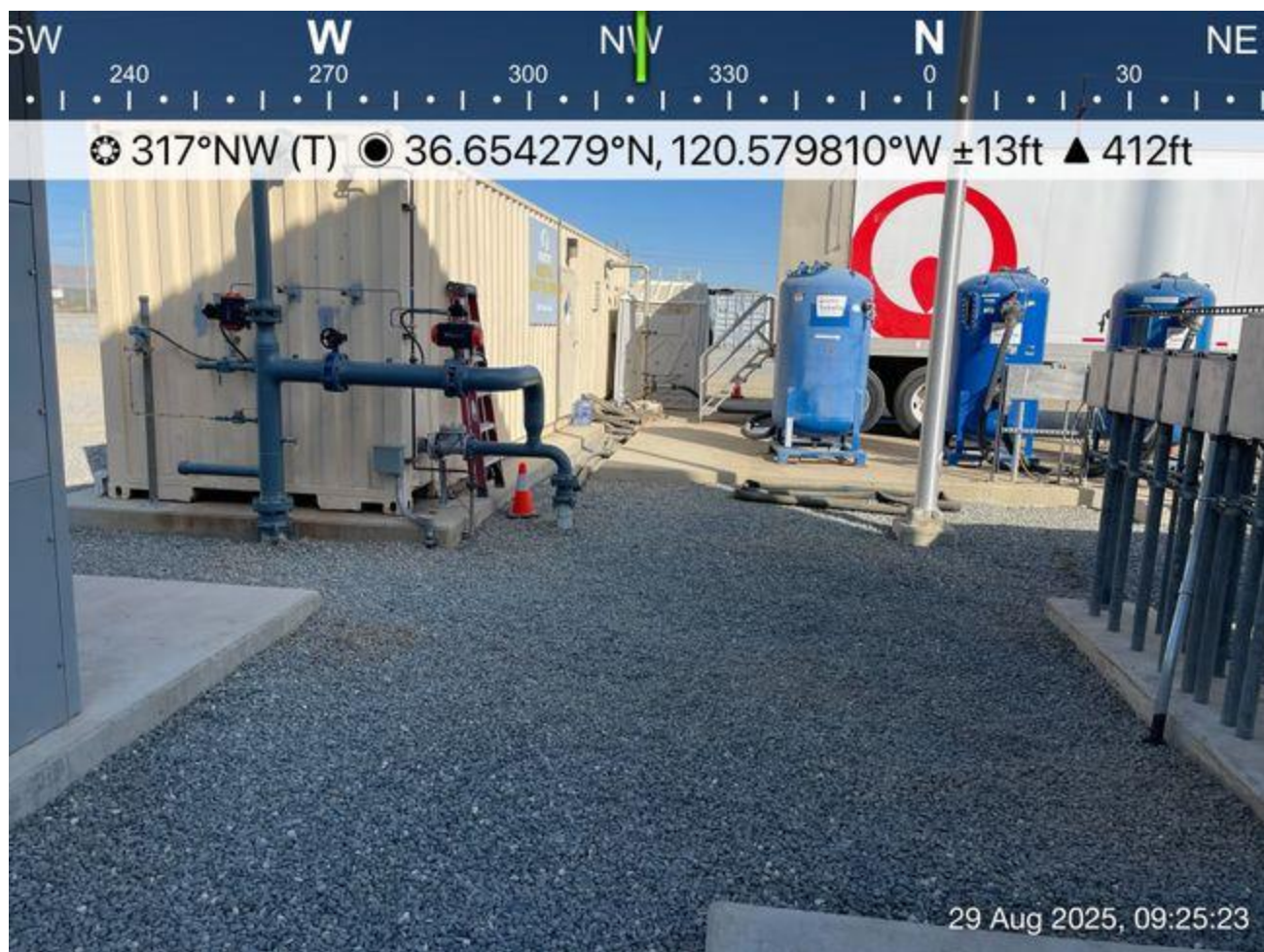
Waterline upgrade worksite and conex, with door closed.
