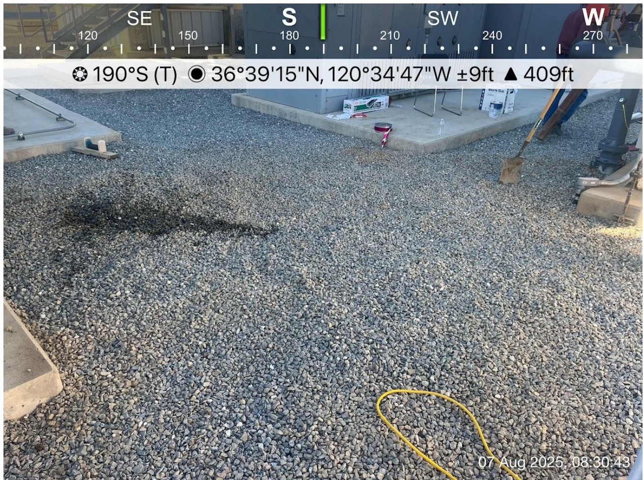
Conduit trench after completion of backfill.
