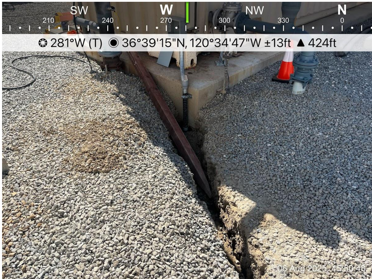
View of conduit trench at end of day with wooden post used as wildlife escape ramp.
