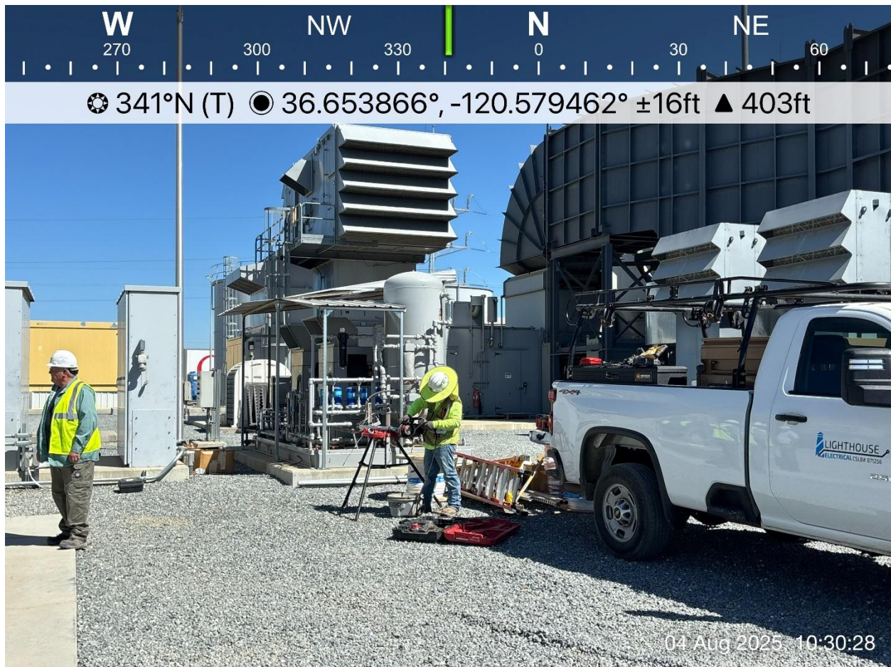
Above-ground utility work.
