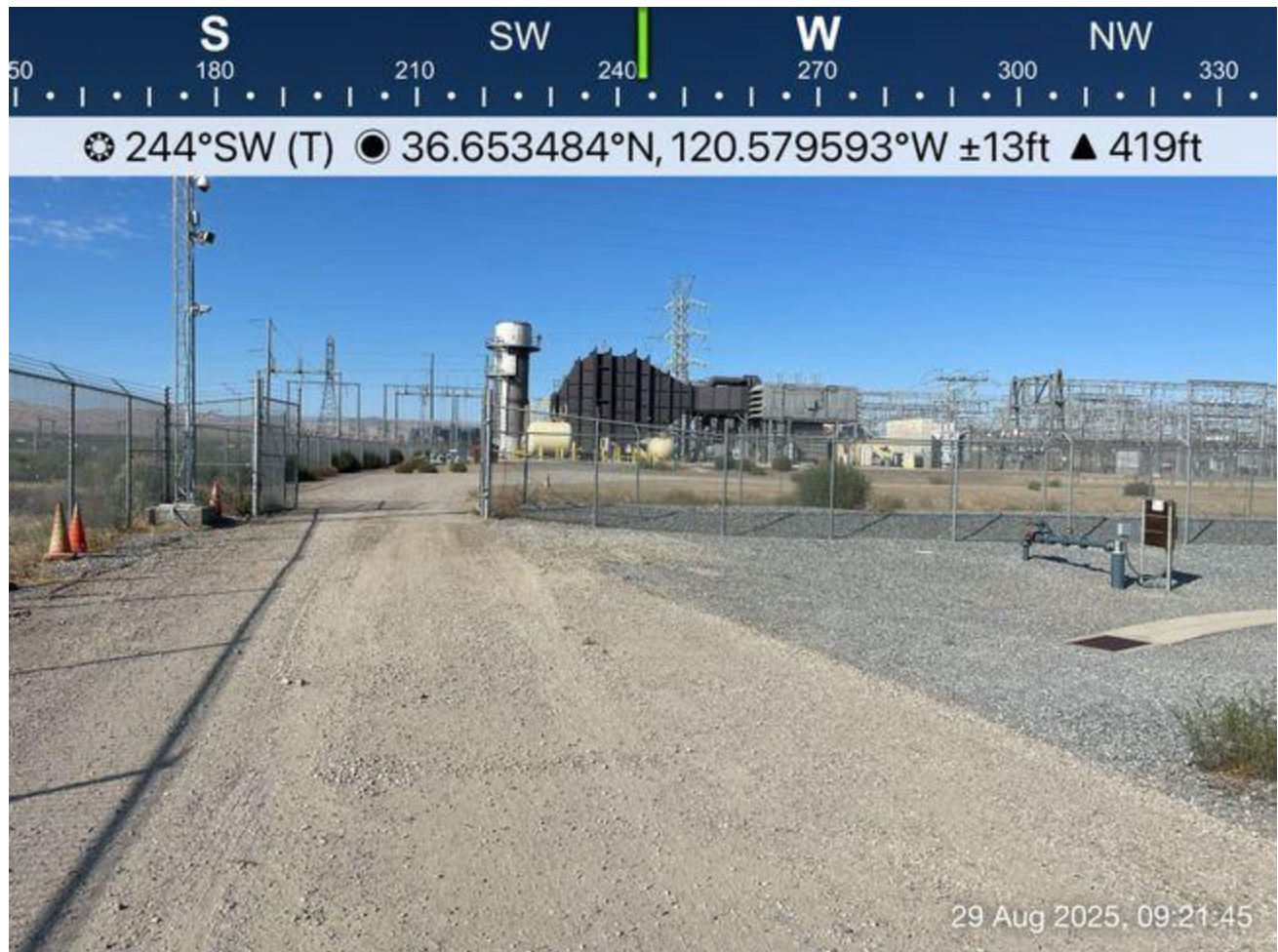
Waterline valve former excavation site.
