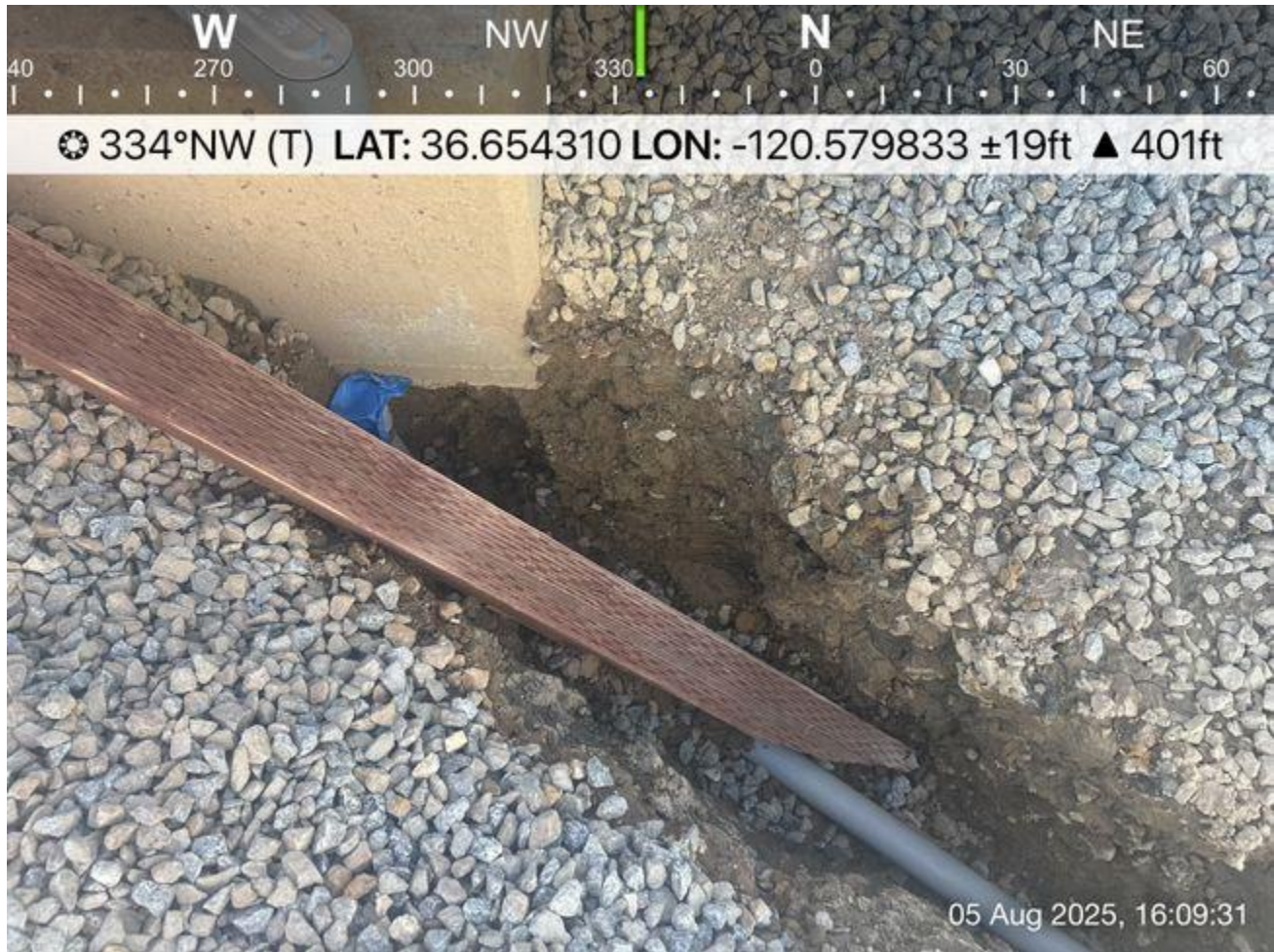
Photo 1: Wooden board used as wildlife escape ramp in trench and conduit capped.
