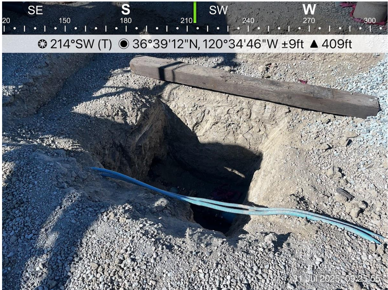
Valve excavation prior to inspection/ work.
