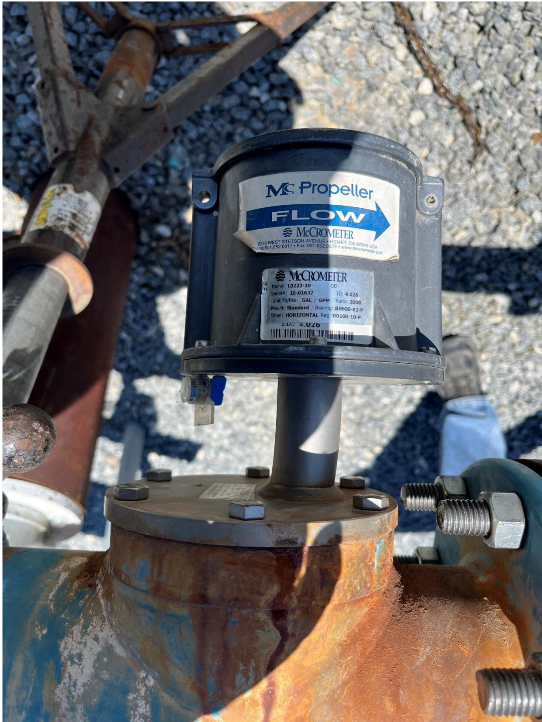
Photograph #7: Existing Flowmeter and check valve removed for test.
