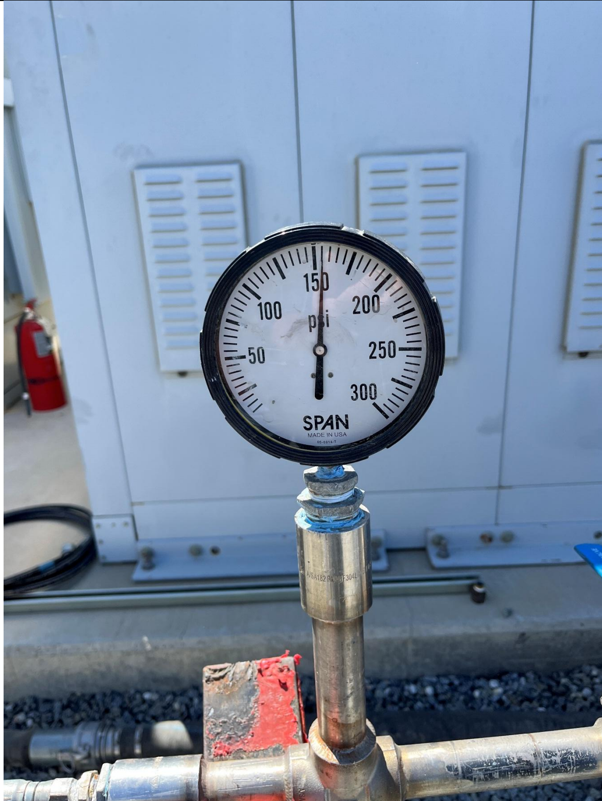
Photograph #1: Line pressure test at start of inspection.
