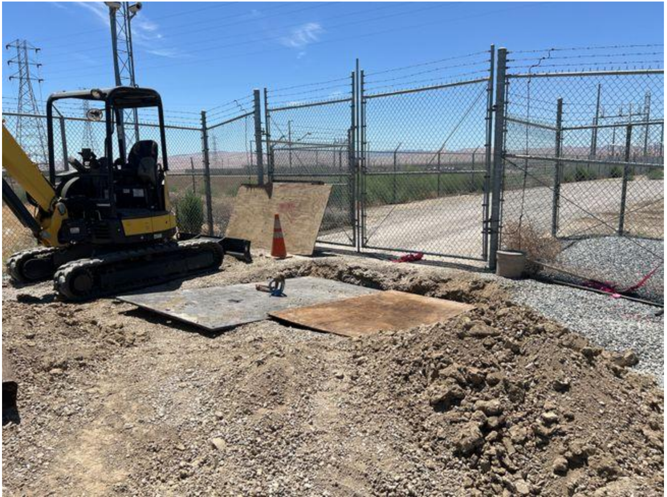
Trench check prior to scheduled work activities.
