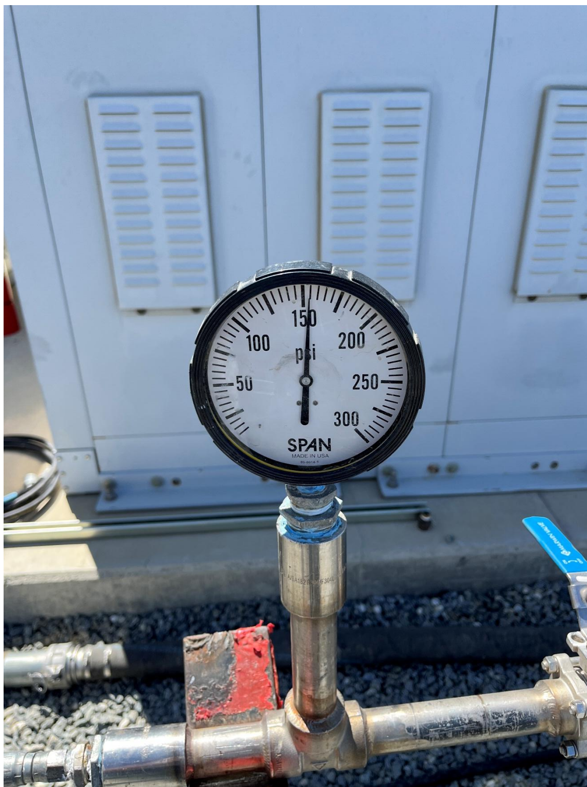
Photograph #2: Line pressure after 30 min. No drop in pressure.
