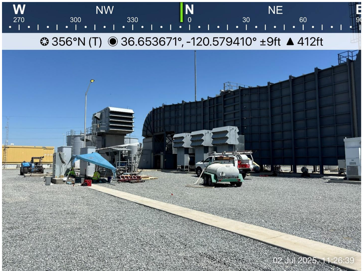
Electrical work overview.
