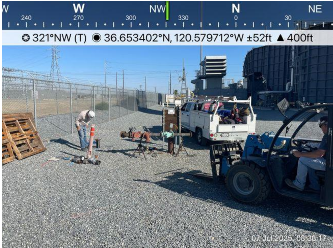
Above ground pipe near the valve excavation was lifted and put on stands for work
