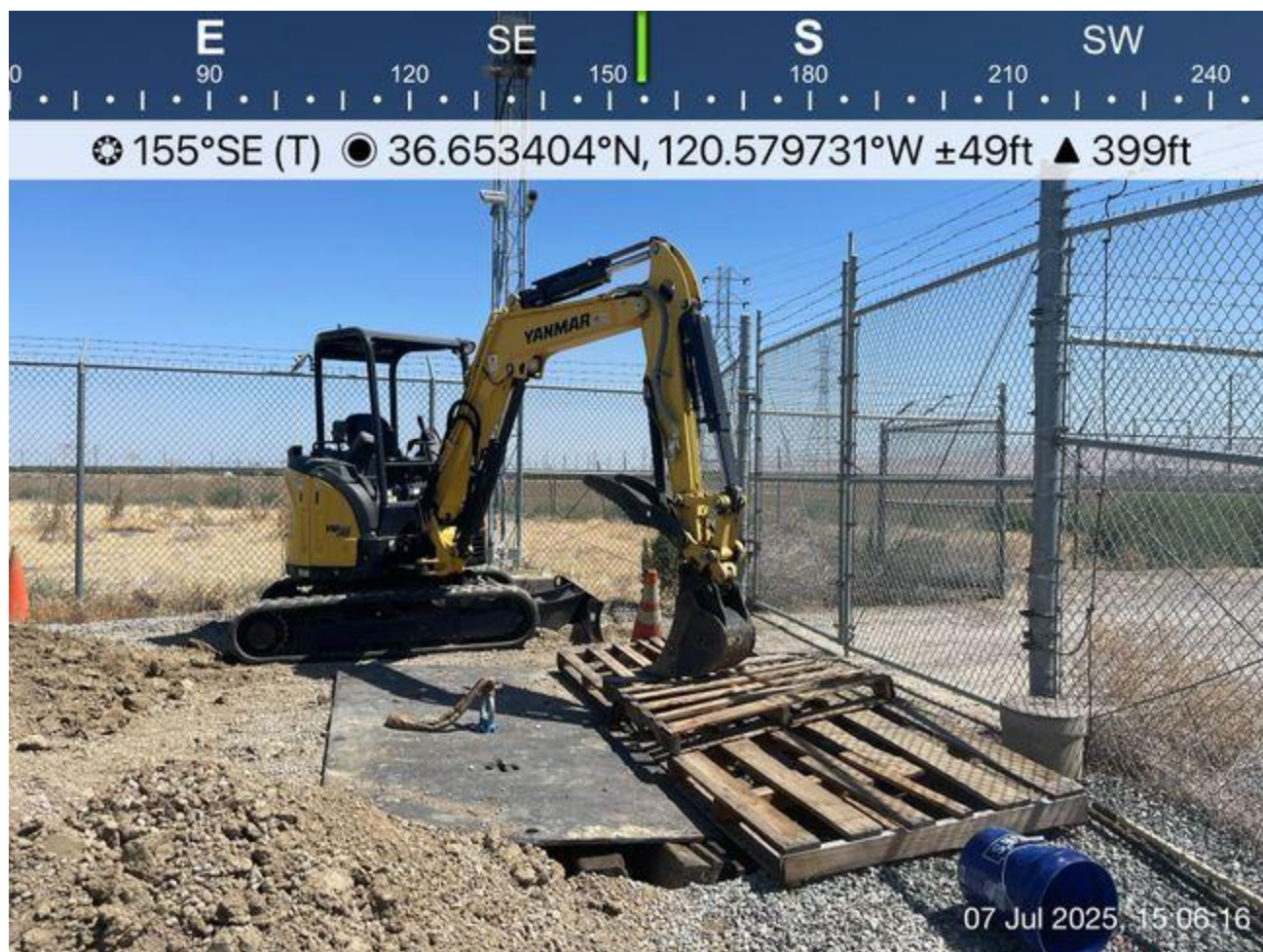
Excavation covered with railroad ties, a steel sheet, and wooden pallets at the end of the day.
