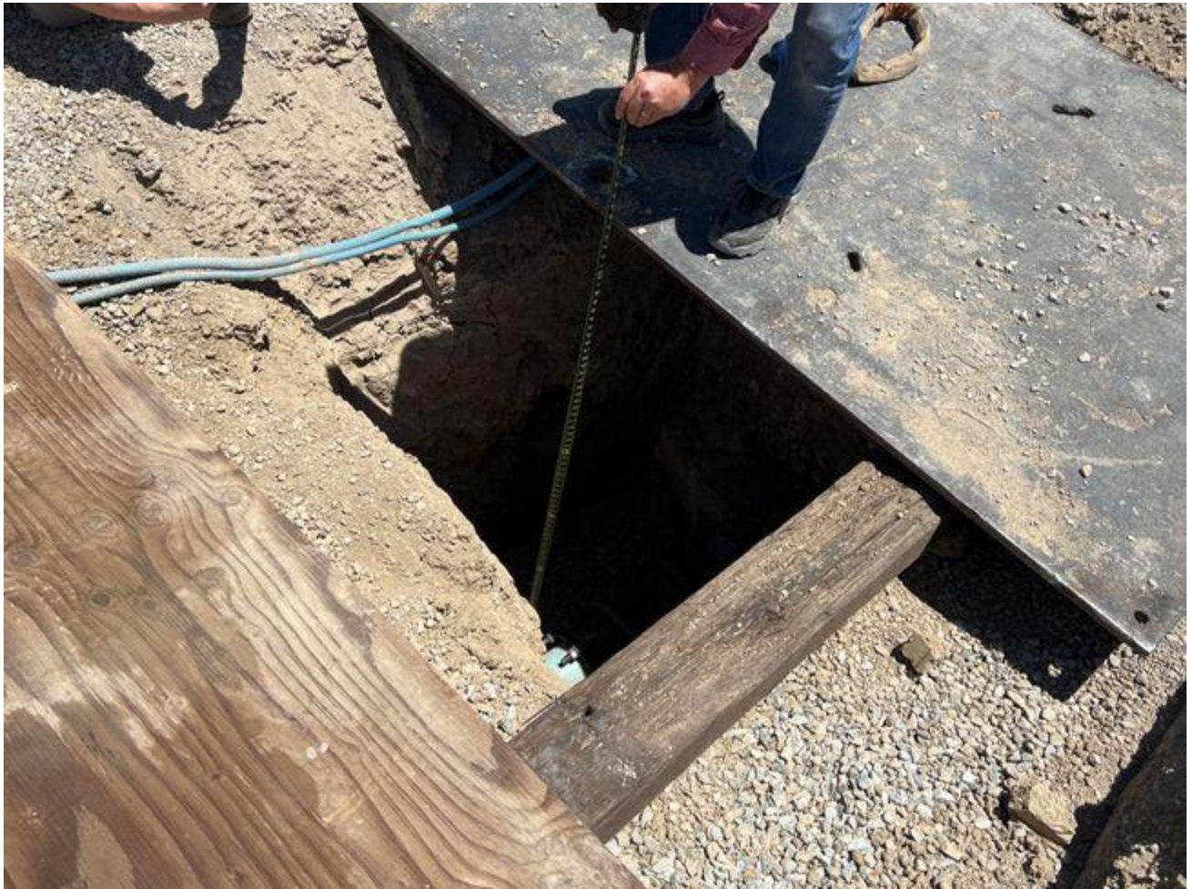
Trench opened with pipe work commencing.
