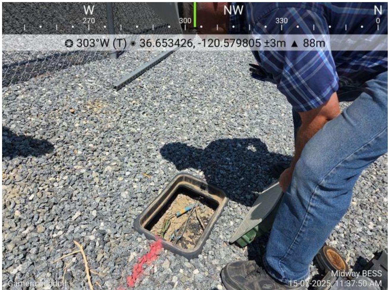
Inspecting splice box
