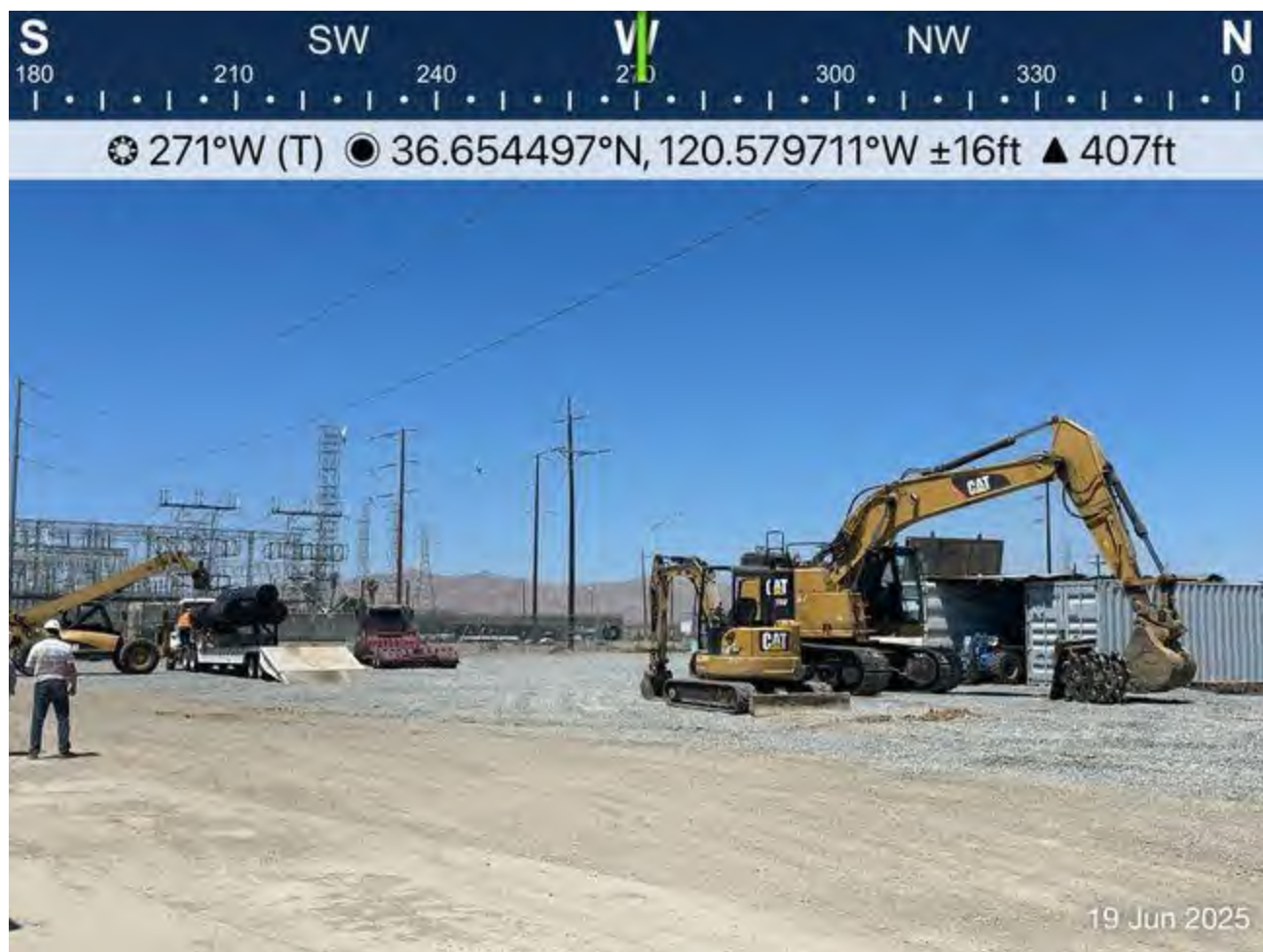
Pond lining delivery and heavy machinery pick up
