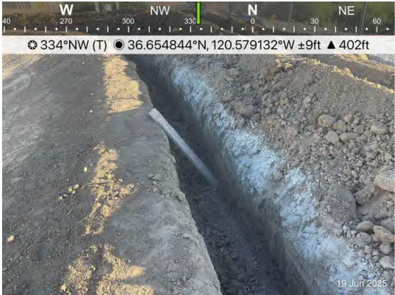
Morning trench check with wooden wildlife escape ramps installed.
