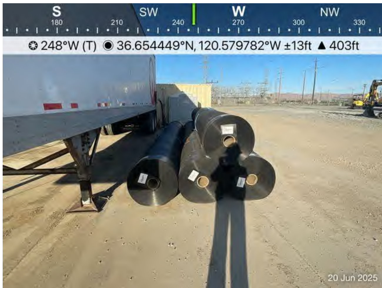
Staged pond liner
