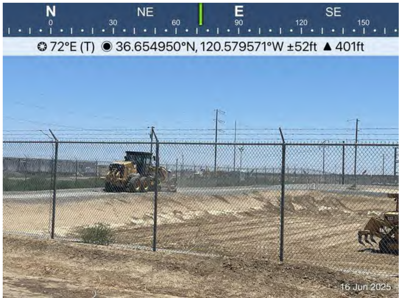
Scraping to remove gravel along the edges of the pond
