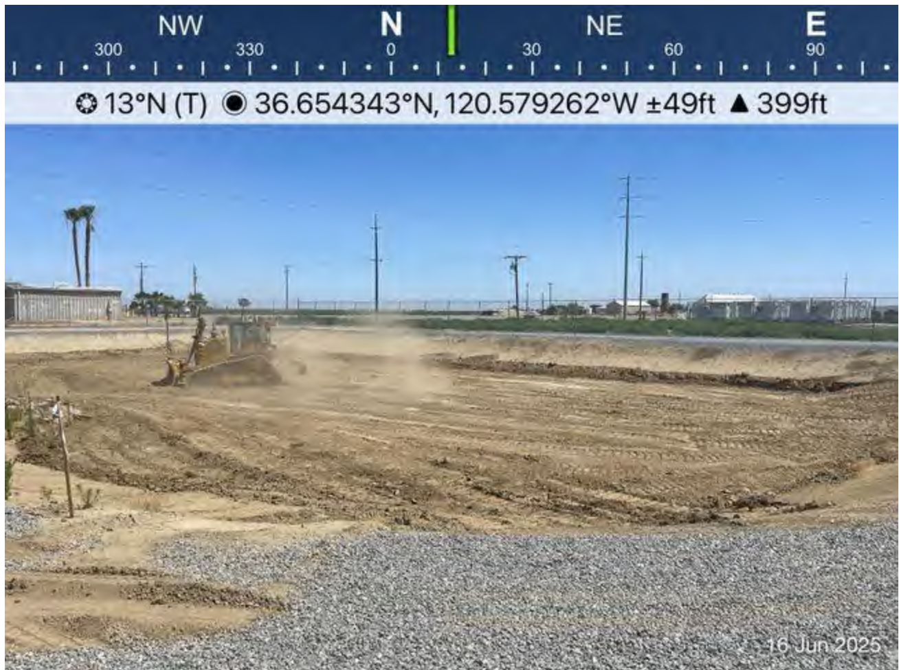
Pond lining excavation
