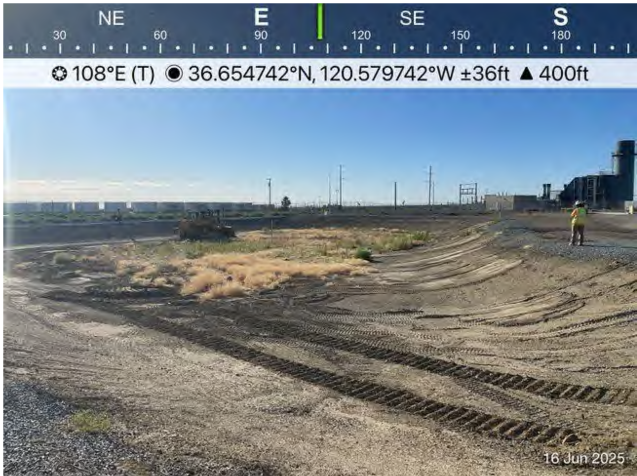
Pond before excavation
