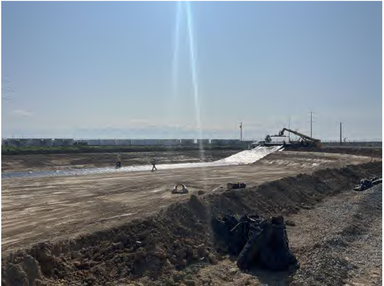
D&E crew rolling out pond lining into the evaporation pond.
