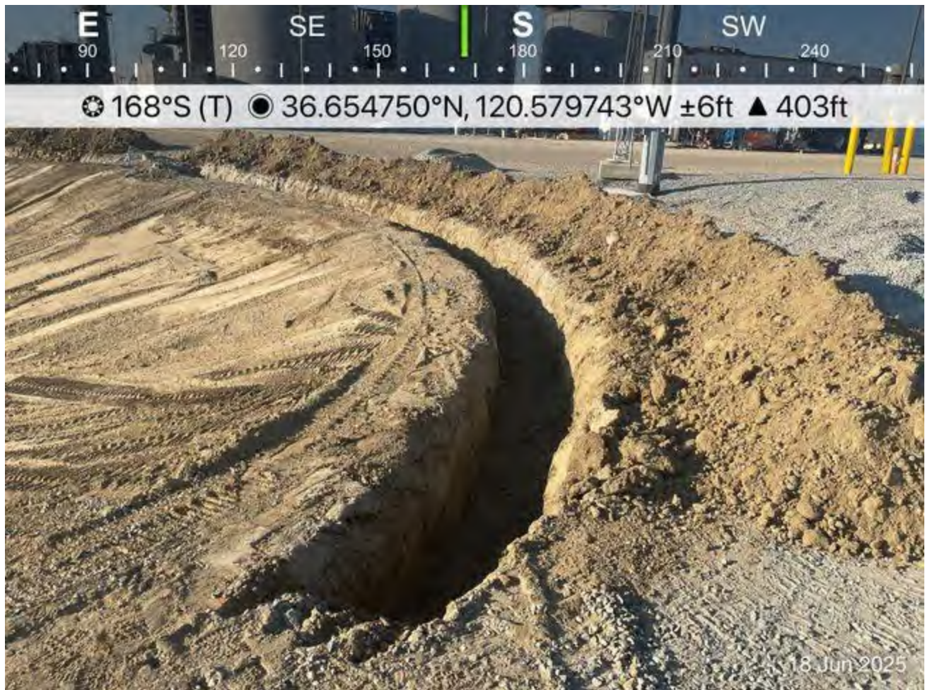
Morning trench check for wildlife
