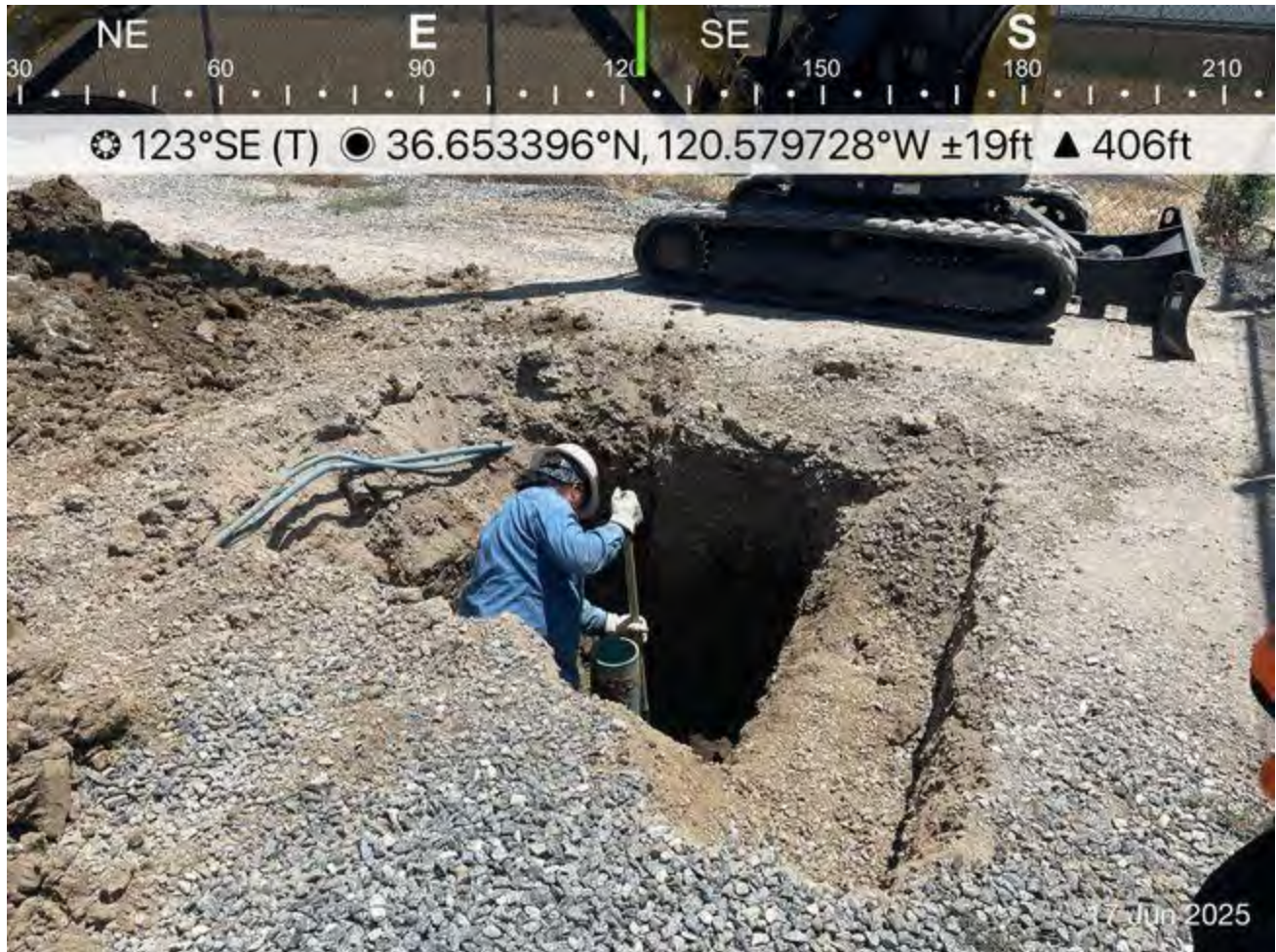
Excavation to water pipeline approx 4 feet deep
