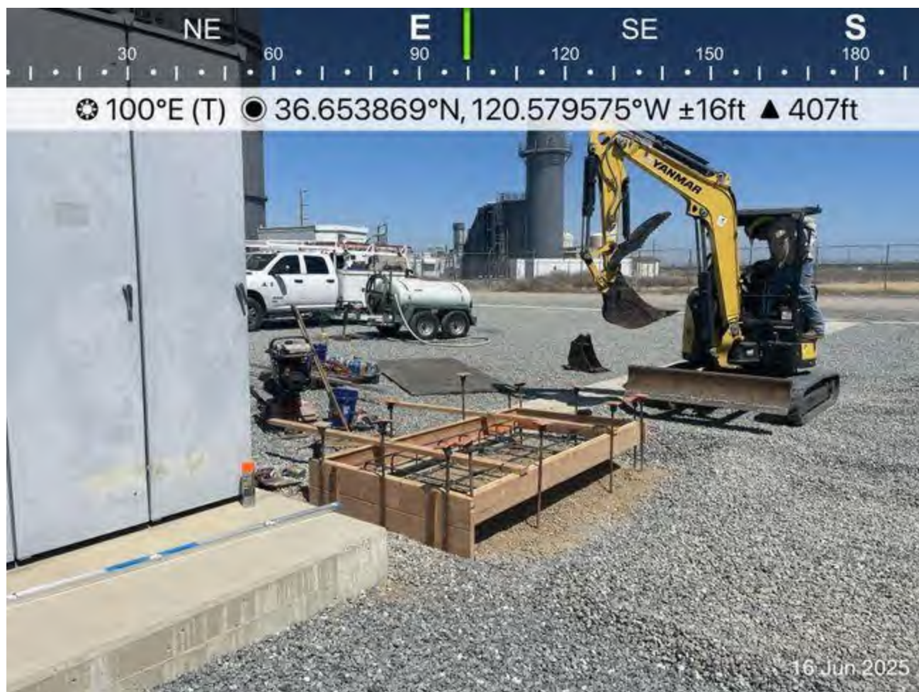
Concrete pour site being cleaned up for the day. Pour will likely occur tomorrow
