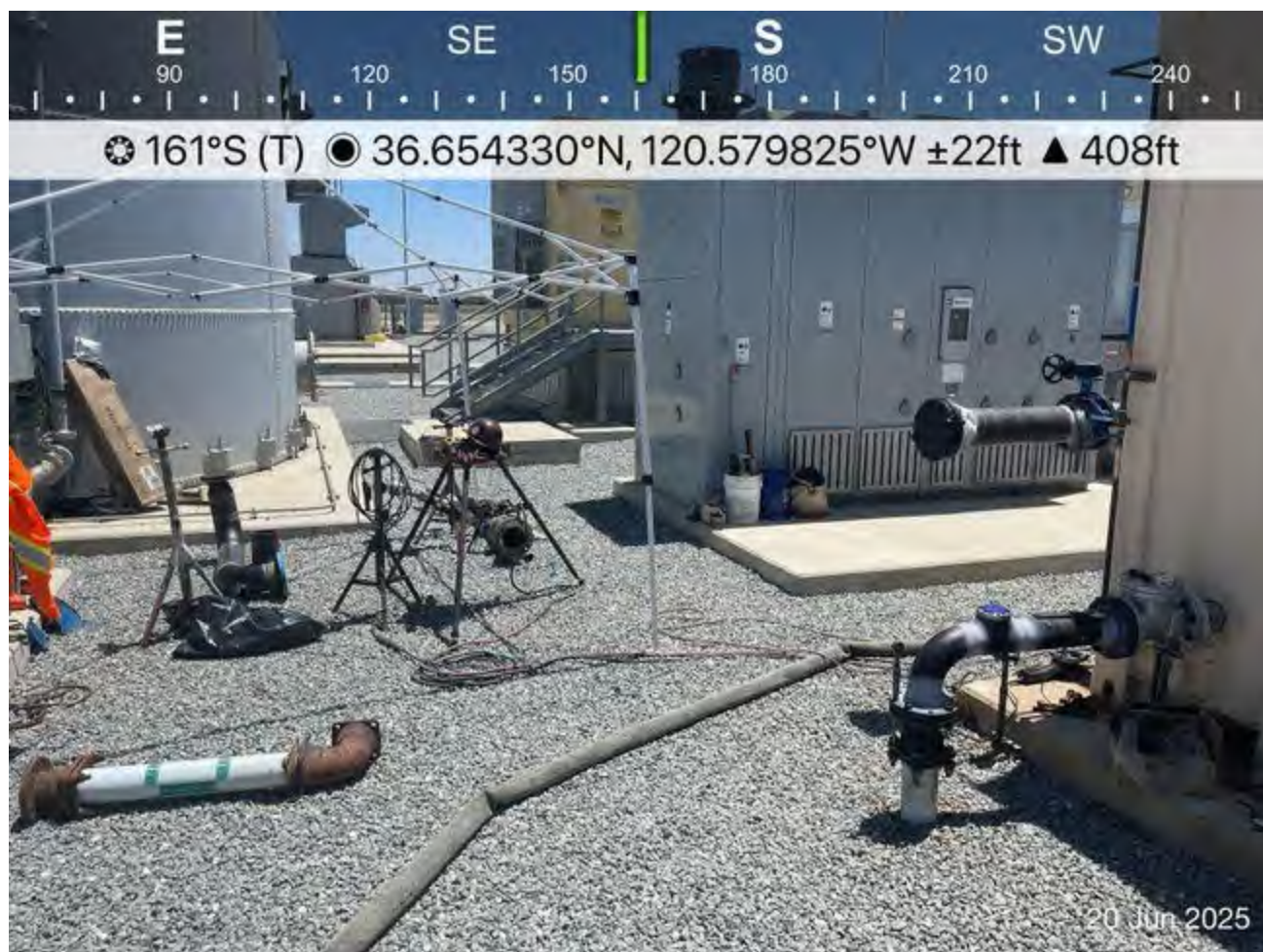
Work site at end of day
