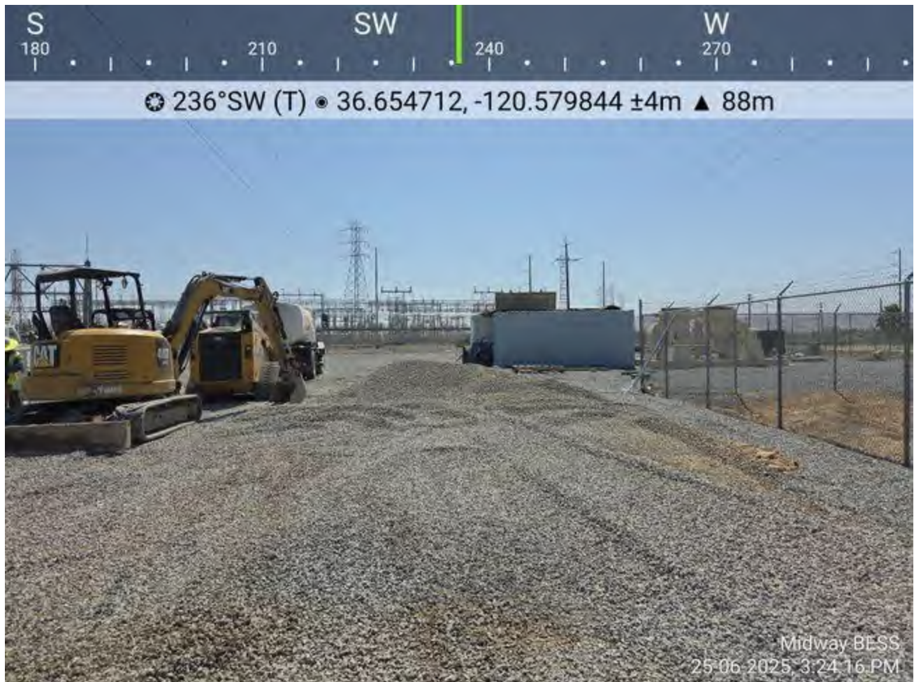
Post-work staging overview
