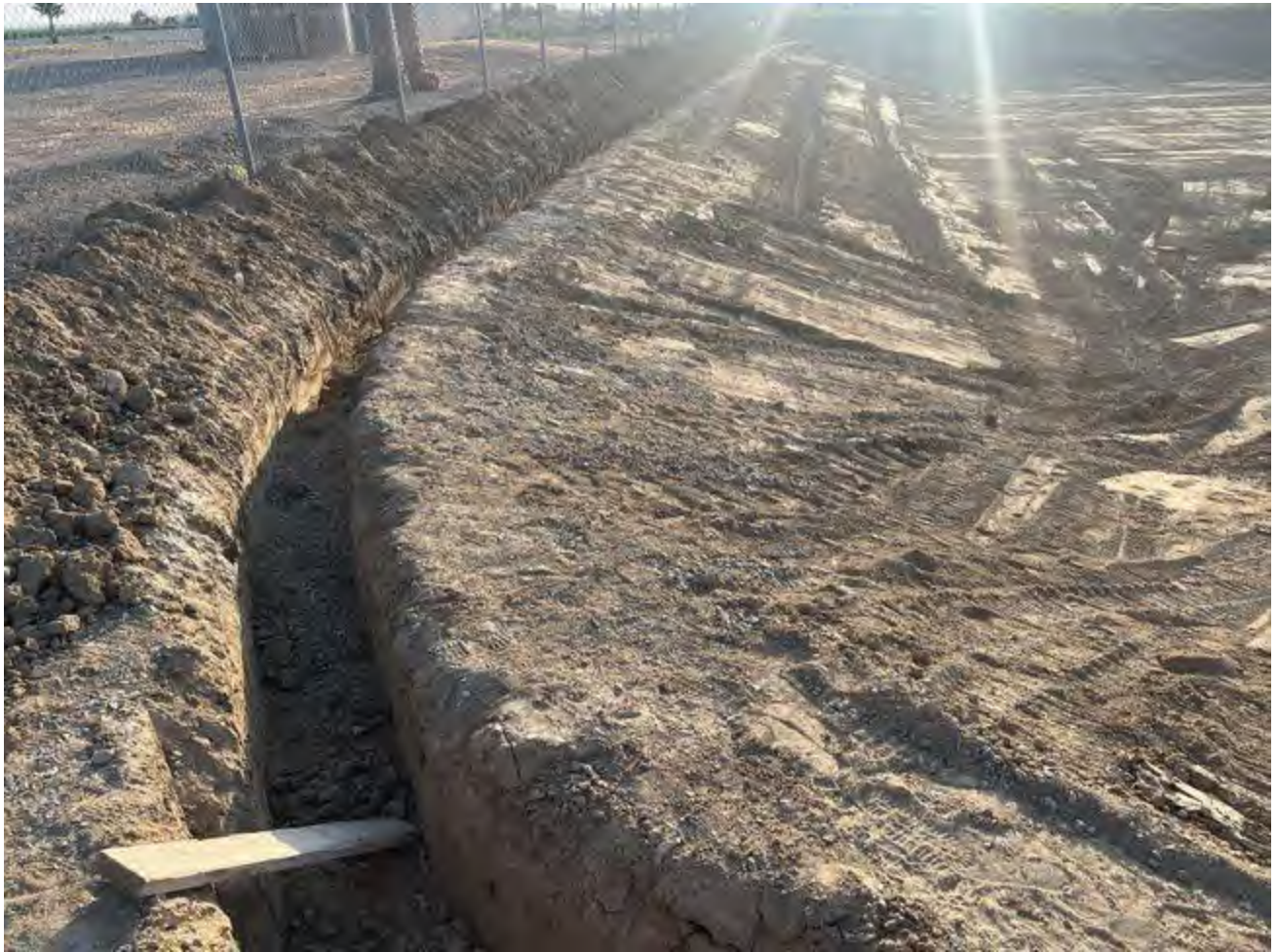
Environmental sweep of work area with adequate wooden plank ramps for wildlife entrapment prevention. No wildlife or environmental concerns observed.
