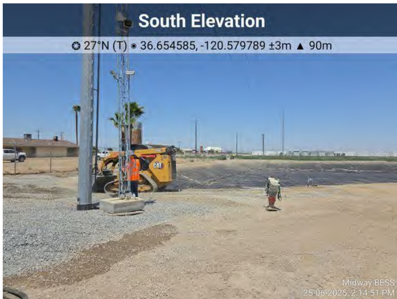
Smoothing gravel over compacted trench
