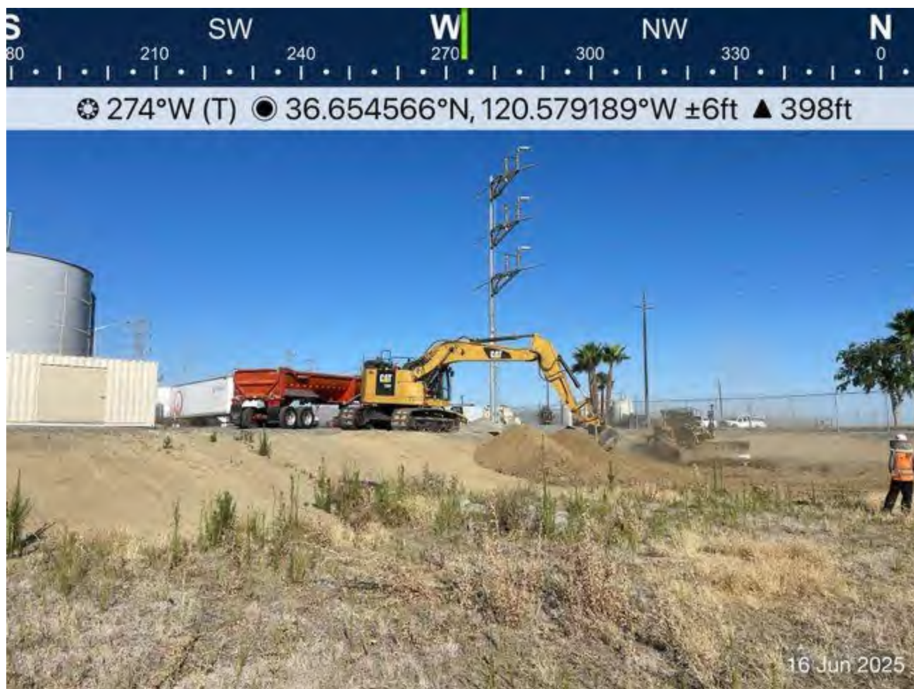
Soil being loaded to be taken offsite.
