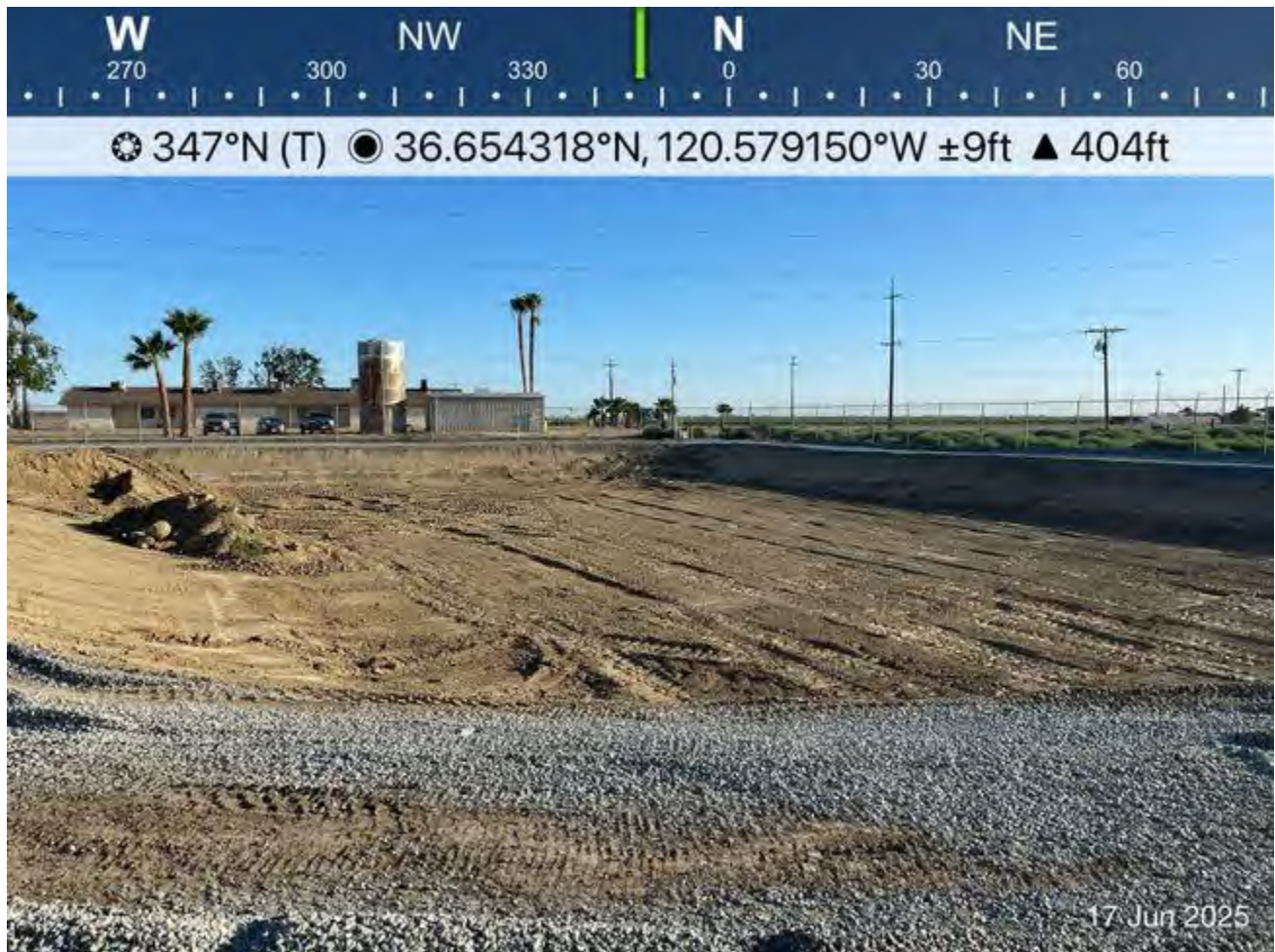
Photo of pond before work begins
