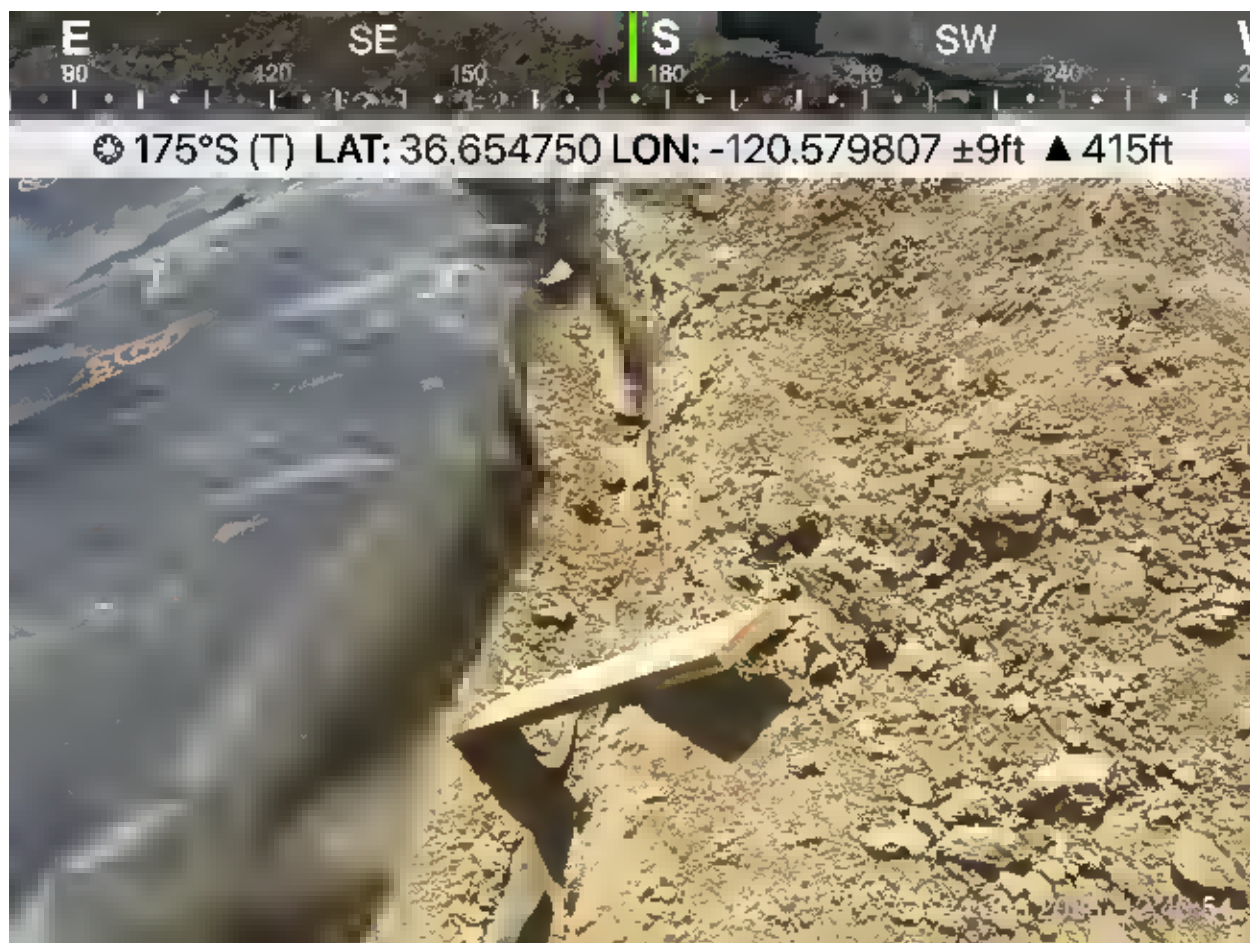
One of three escape ramps that were added to the trench once work was complete, facing south. June 24, 2025.
