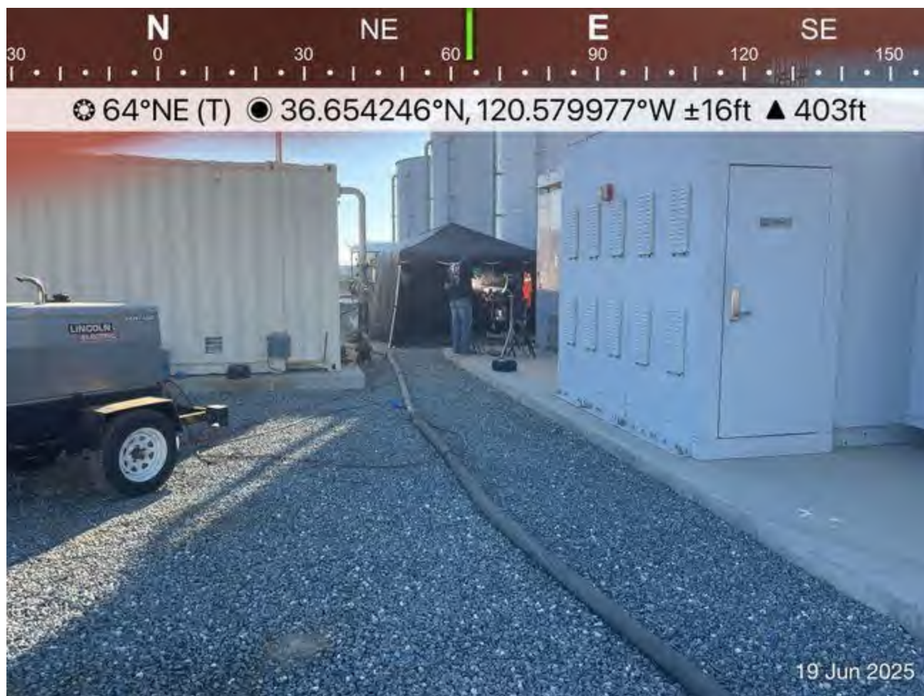
Welding work on pipes
