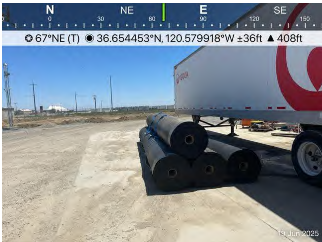
Pond lining staged on worksite
