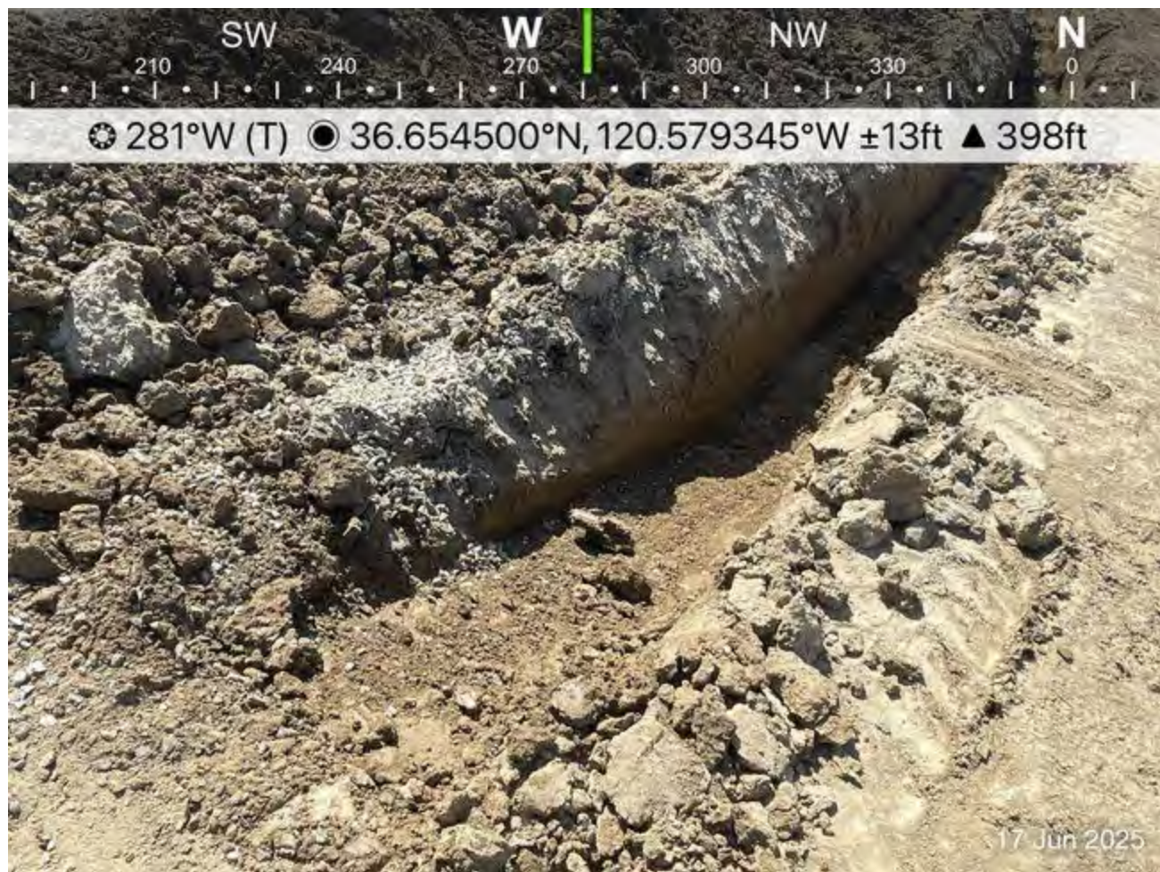
Earthen wildlife escape ramp in each trench
