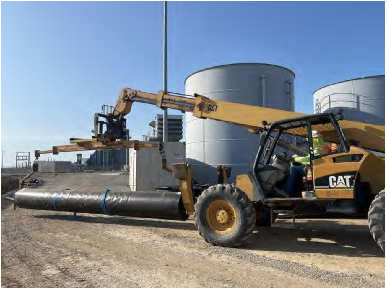
Pond liner rolls relocated using a forklift with special attachment.
