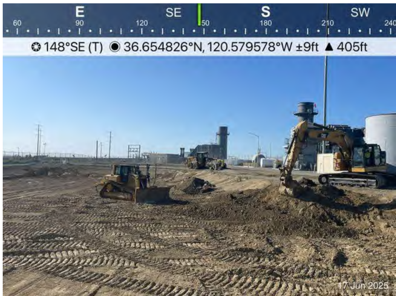
Crews scrapping up gravel along the outside of the pond to clear for trenching
