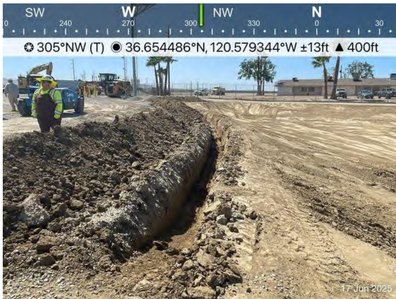
Trench at end of work day
