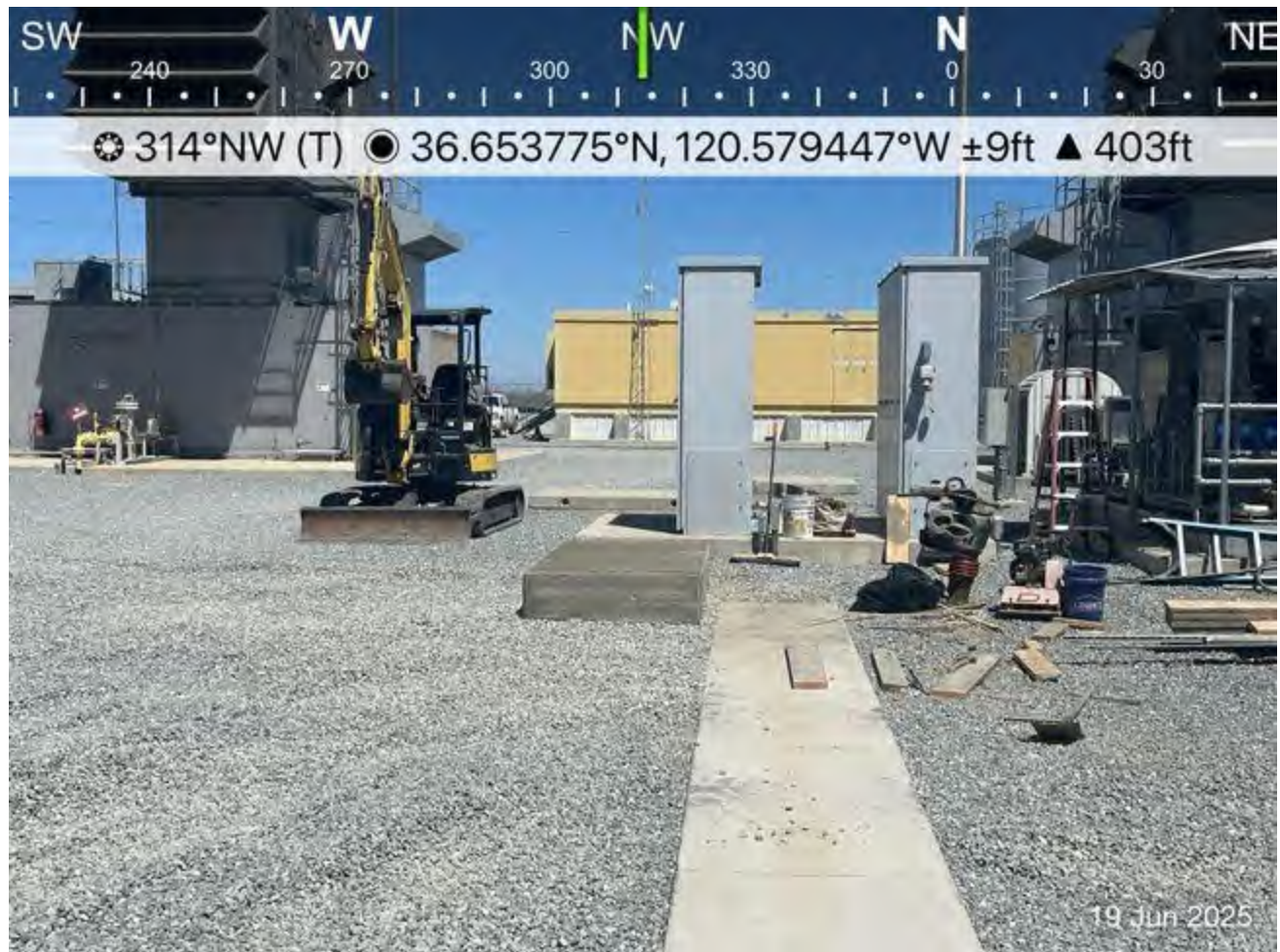
Wooden form removed from concrete slab after yesterdays concrete pour
