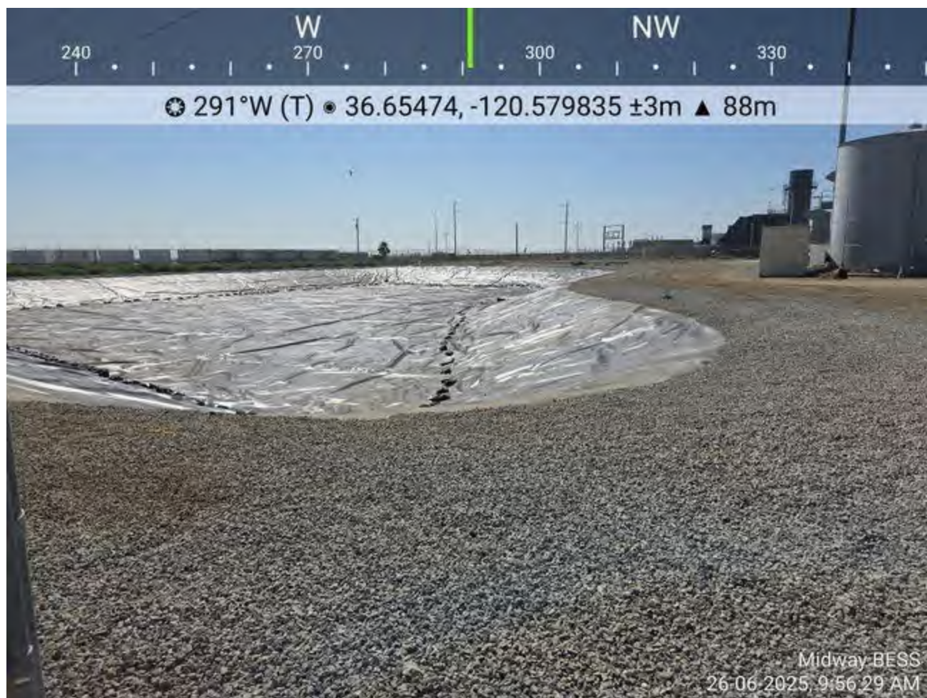
Pond liner installed
