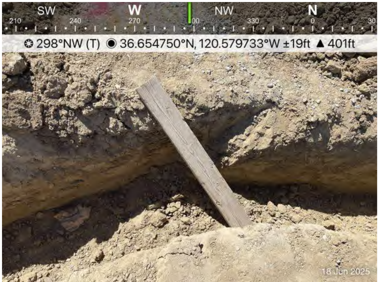
Wildlife escape ramps placed every 200ft in trench
