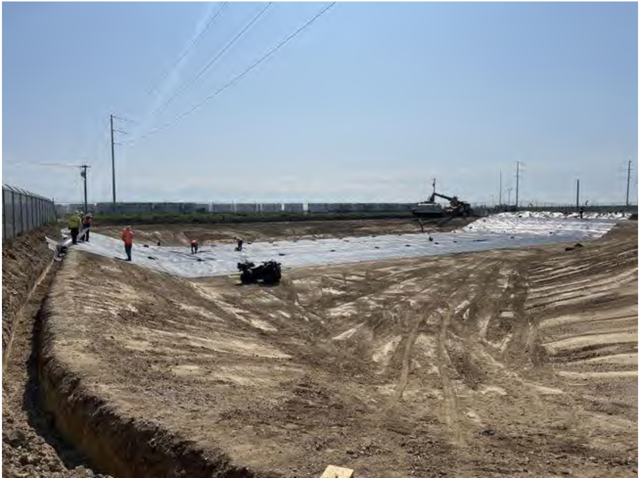
D&E crew continuing pond lining work activities.
