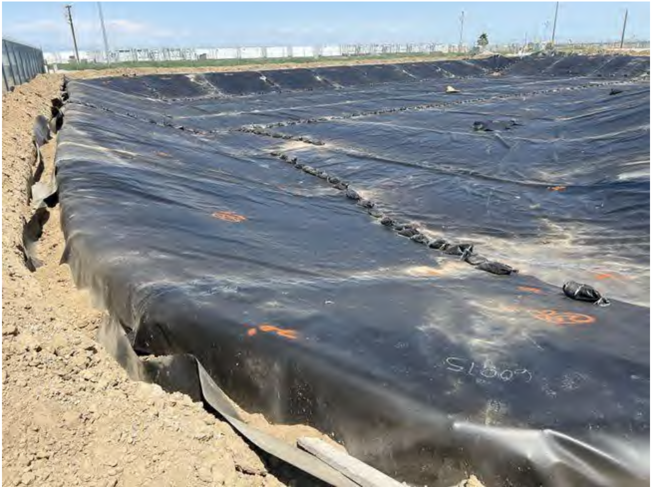
End of day with no compliance concerns. Adequate wooden ramp visible in foreground.
