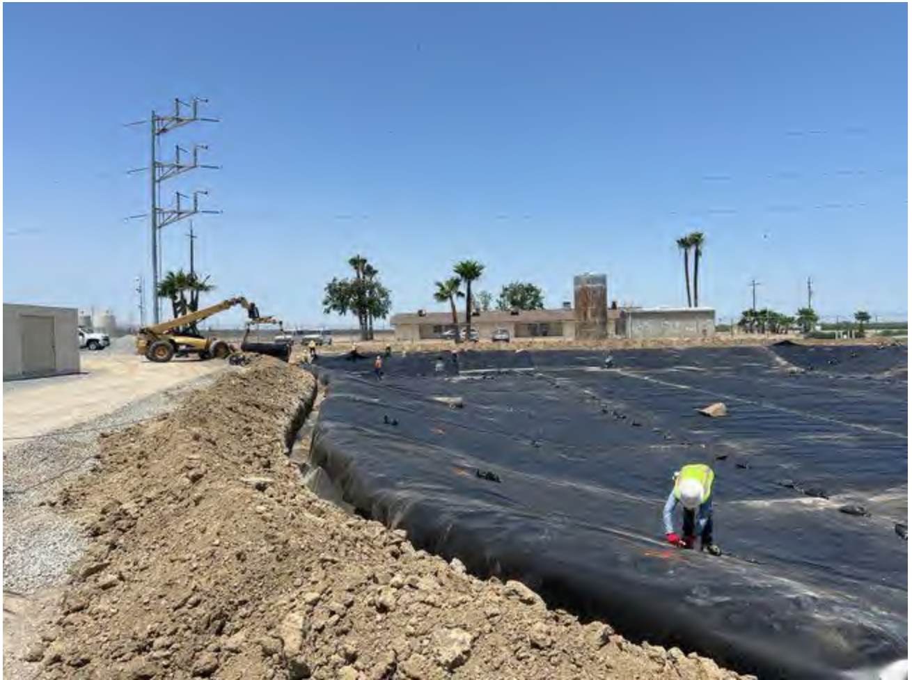
Pond lining work continued.
