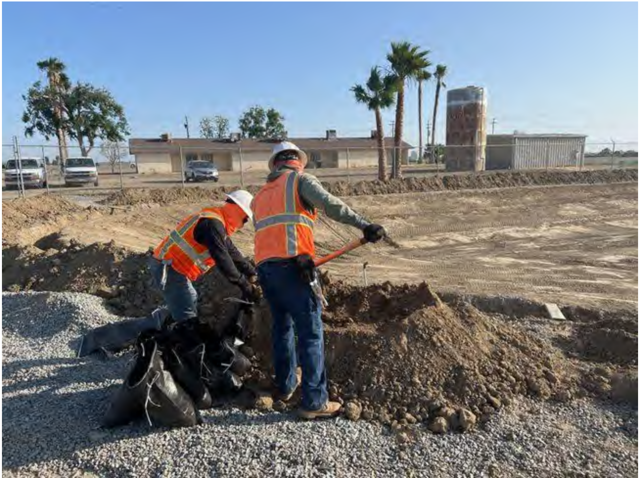
D&E crew preparing bags of dirt for securing pond liner during installation. Dirt was used from stockpile around pond edge utilizing hand tools.
