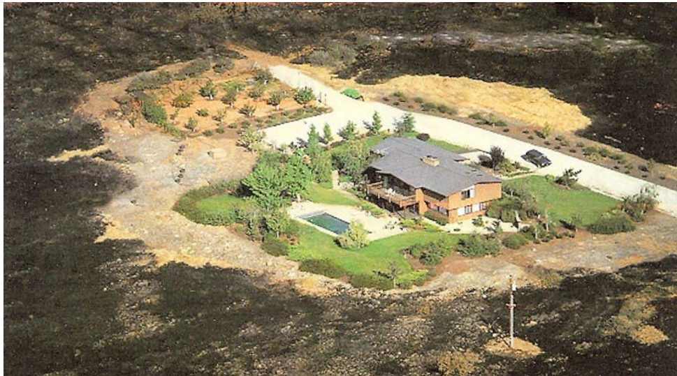
Figure 1. Home designed to withstand wildfire damage through wildfire resistant landscaping and engineered building practices. Source: Department of Energy. 1
