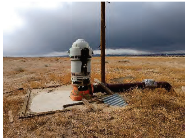
Photo #28 View of an inactive water well pump located on the western side of Willow Avenue on Tract 3.
