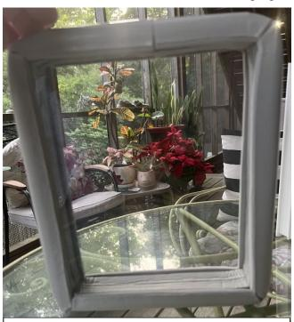
Above: a 3 glazing layer unit is sealed by the fold-down lip front and back. Two such units friction-fit into a framed opening to create an R6.6 fixed window. The exposed grey foam acts as a gasket sealing against trim inside and out, caulked at the perimeter to provide a water-&-air-tight seal. Emergency egress & ventilation are provided by doors with screens.
