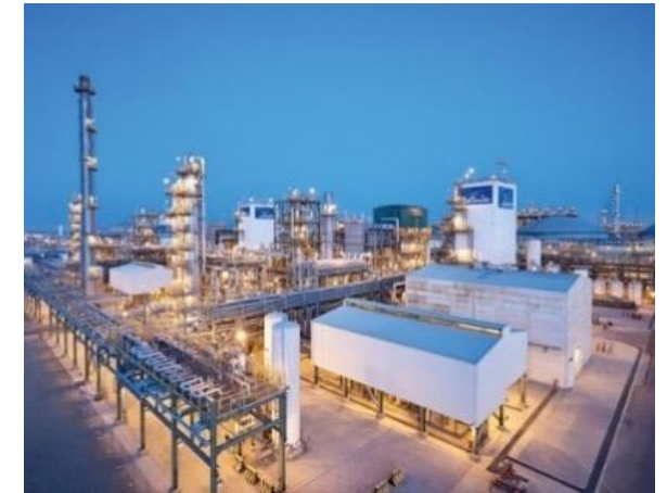
H 2 plant featuring various technologies
