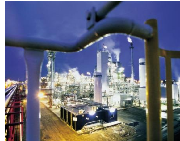
Linde steam reformer
