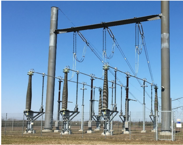
Figure 5 - Example HV Cable Terminations transition with overhead line.
