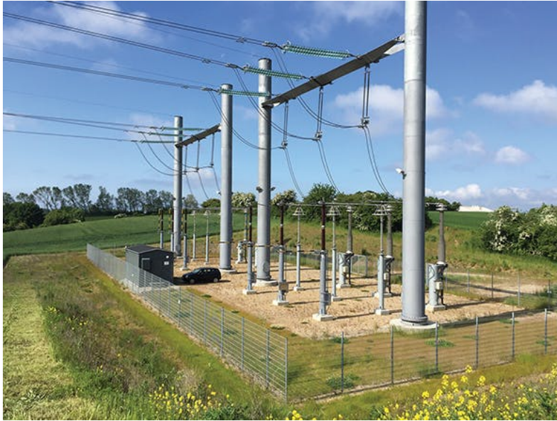
Figure 11 - Example 400kV Transition Compound (Source: Reimagining the Grid | T&D World )
