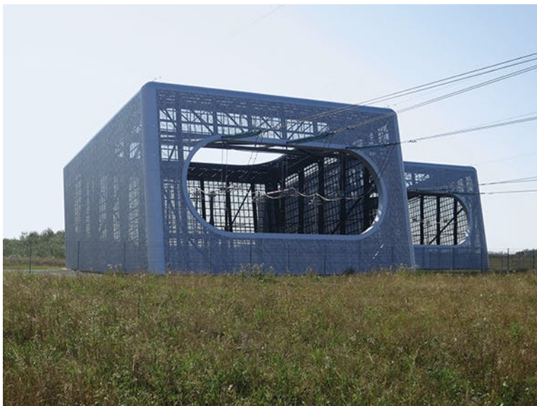
Figure 14 - Example Fenced Transition Compound (Source: Reimagining the Grid | T&D World )
