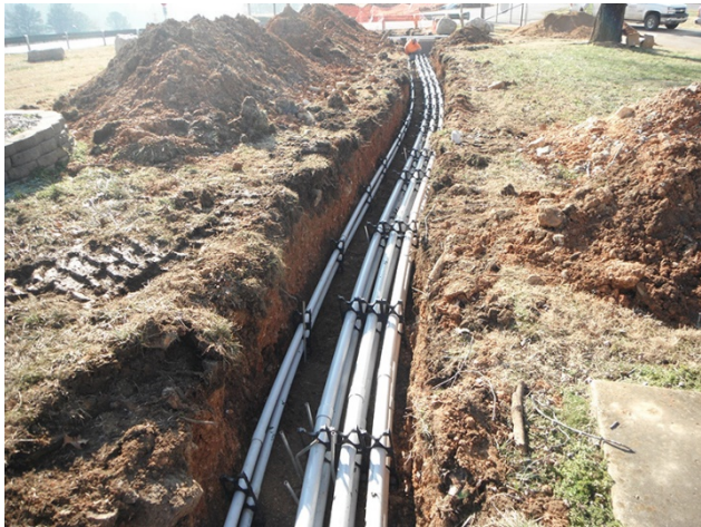
Figure 3 - Example Duct Bank in Open Cut Trench (Source: Wappapello Lake Duct Bank Project)
