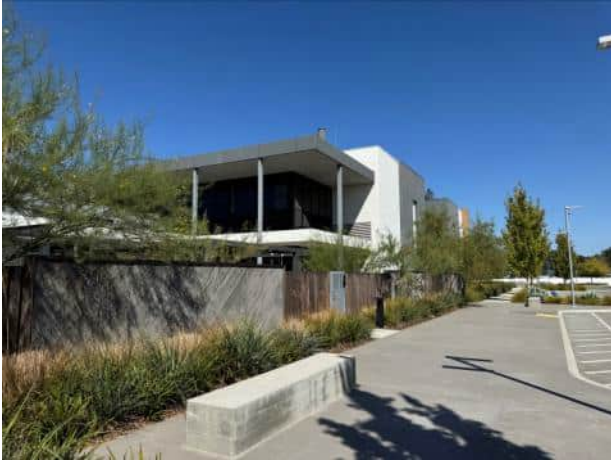
37. View of the exterior of the subject property
