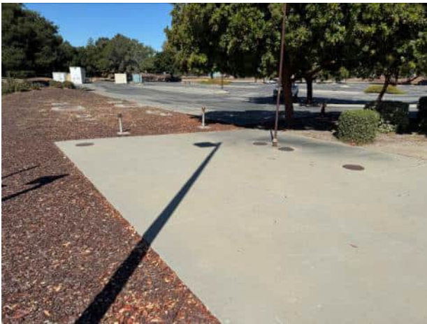
33. View of the UST installation
