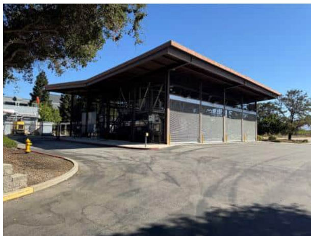
30. View of ammonia storage
