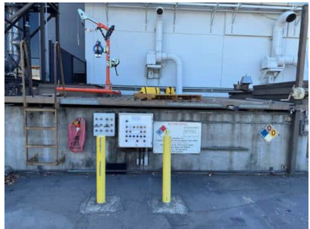
18. View of waste storage vaults
