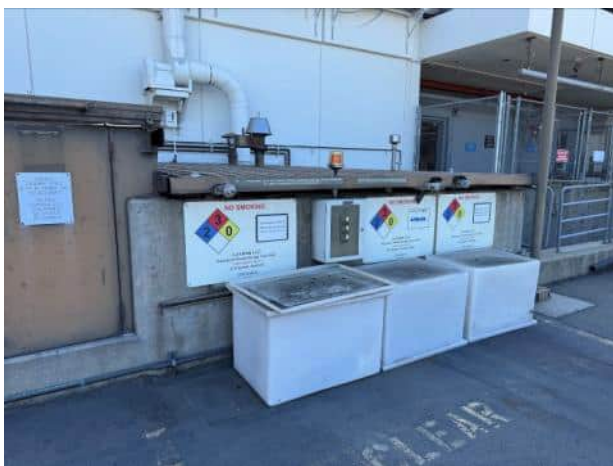
21. View of waste storage vaults
