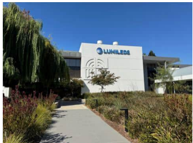
36. View of the exterior of the subject property
