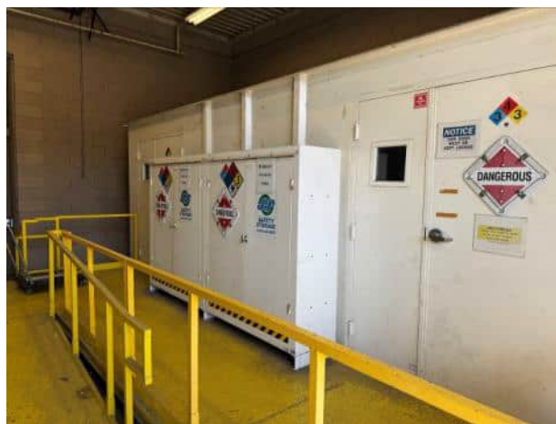
22. View of chemical storage
