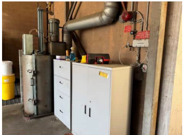
6. View of the hazardous waste storage area
