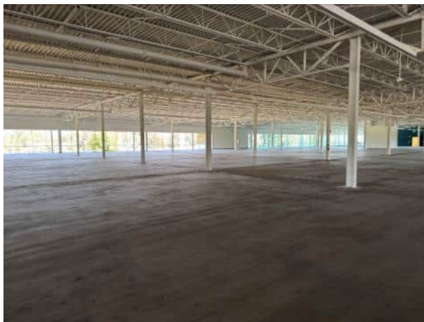
3. View of the interior of the 350 Building
