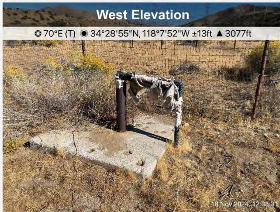
29. Groundwater well located on APN 3056-015-008; current operational status unknown.
