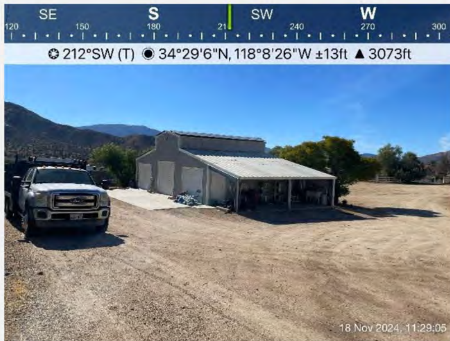
21. A metal outbuilding located near the residential structure on APN 3056-019-026. Access to the interior portions of the structure was not provided during site reconnaissance.
