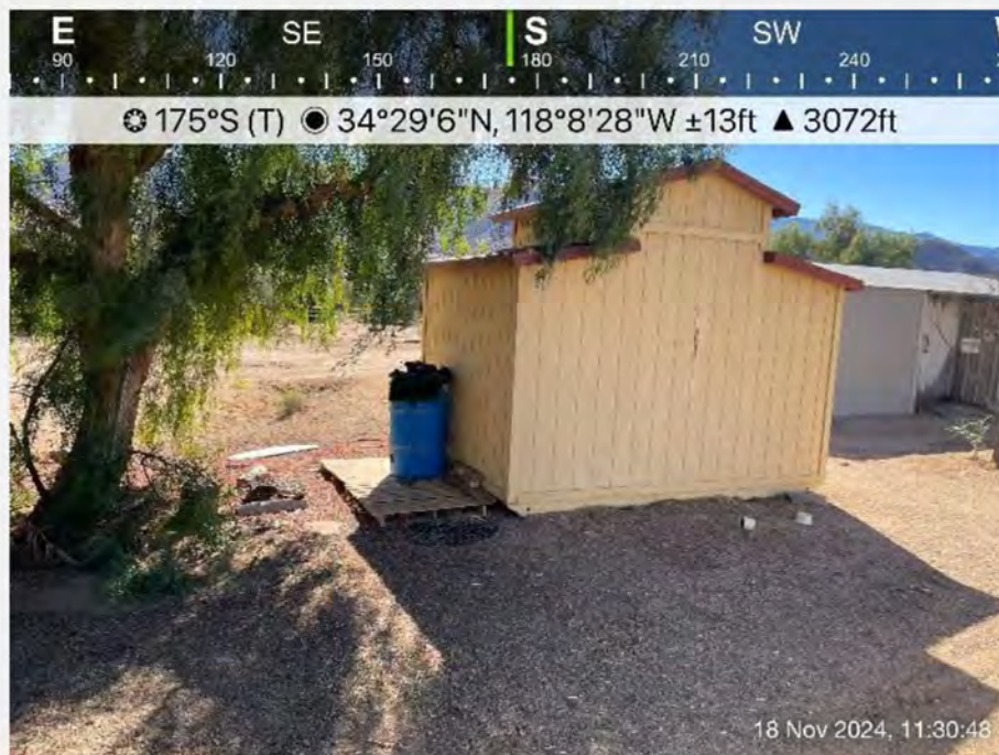
22. One of three outbuildings observed adjacent to the residential structure on APN 3056-019-026.
