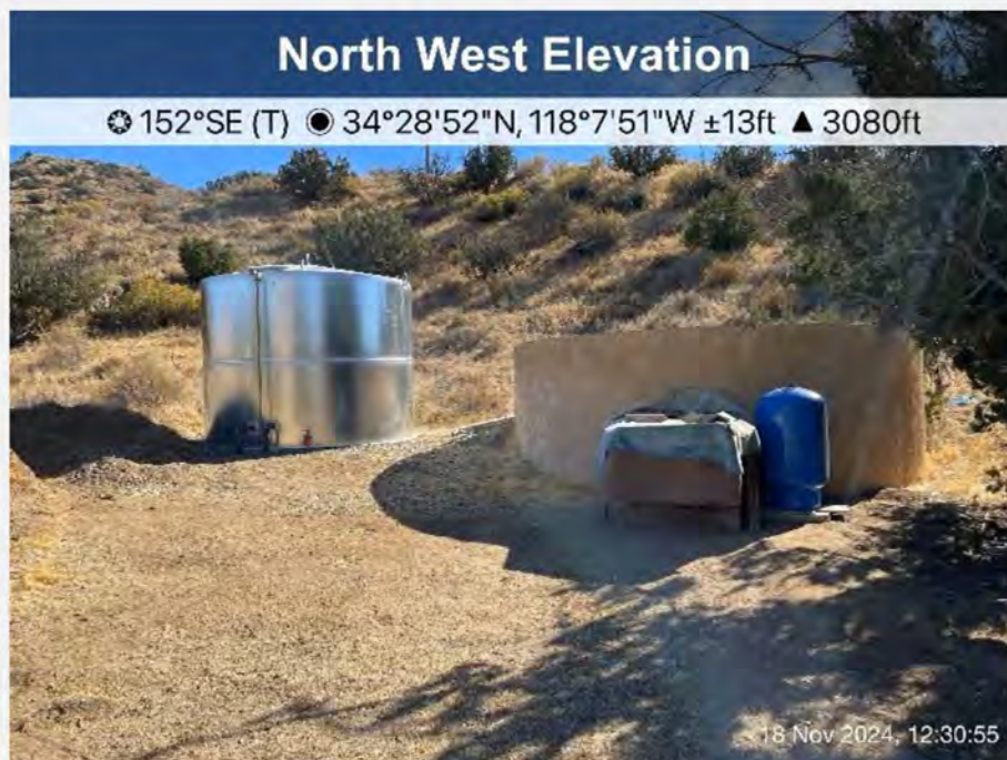
28. Groundwater well located on APN 3056-015-008; assumed to provide potable water to the residential structure located approximately 200 feet southwest of the well.
