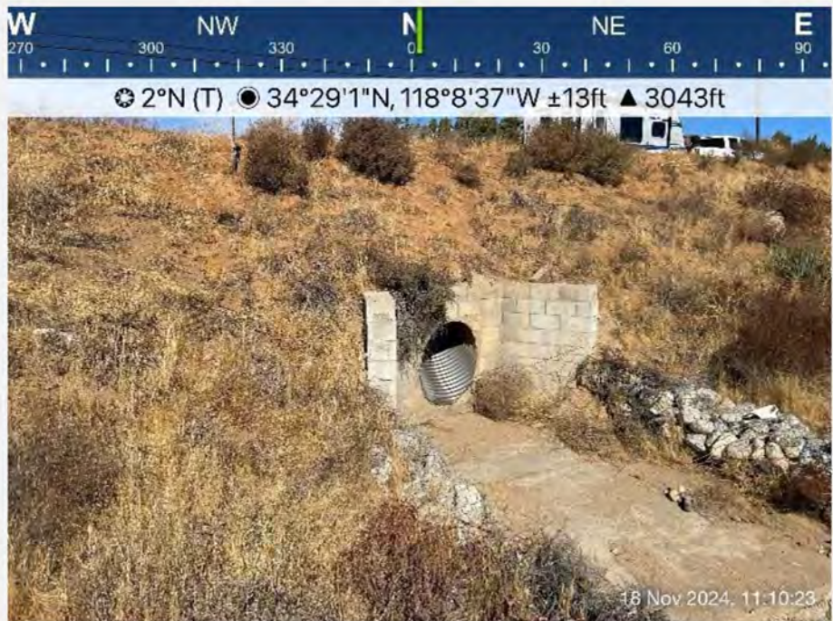
32. Culvert flowing from the northern portions of the subject property below Soledad Canyon Road onto the southern portion of APN 3056-019-040.
