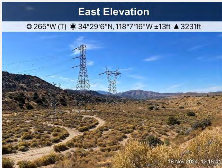
15. Road crossing APN 3056-015-008 and 3056-015-023 providing access to electric transmission lines.
