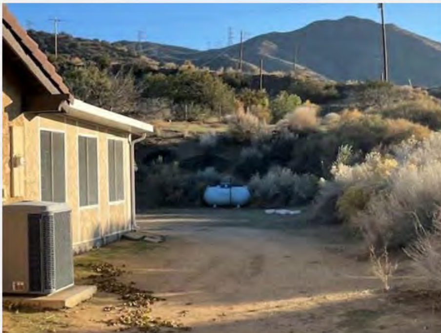
40. One 200-gallon propane tank located adjacent to the residential structure on APN 3056-015-008.
