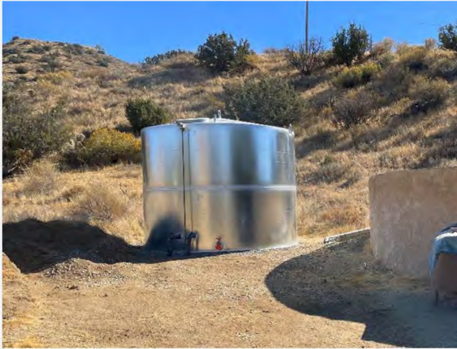
35. The open-air cistern on APN 3056-015-008, located adjacent to one of the two groundwater wells. The cistern was approximately 16 feet across and 6 feet deep; also pictured is a 5,000-gallon water storage tank.
