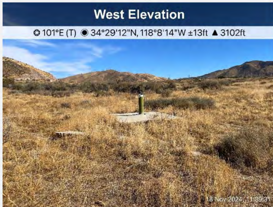
27. Groundwater well located on APN 3056-017-021; power has been disconnected from the pump and no above ground piping was observed.
