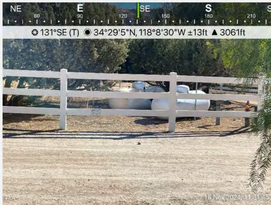
39. Two 150-gallon propane tanks on the north side of the residential structure on APN 3056-019-026.
