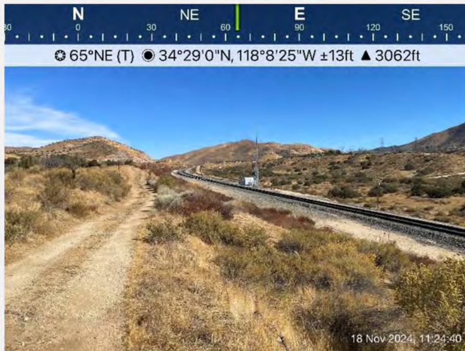
14. Typical access road crossing APN 3056-019-040 providing access to the railroad right-of-way; similar roads cross APN 3056-017-020 and 3056-017-021.
