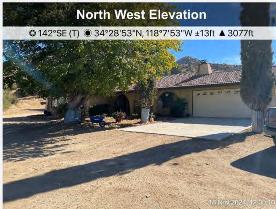
16. Residential structure on APN 3056-015-008. Access to interior spaces of the structure was not provided during site reconnaissance.
