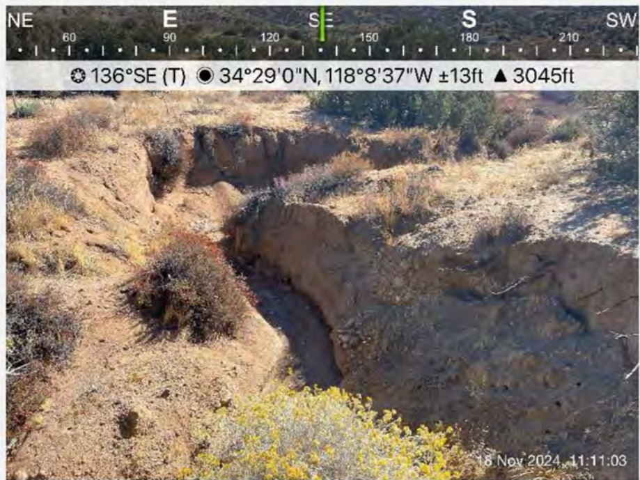
31. Dry ephemeral stormwater drainage ditch on APN 3056-019-040, draining the northern portions of the subject property beneath Soledad Canyon Road and the railroad.
