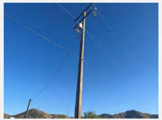
**Photograph 18.** A pole-mounted transformer, likely providing power to the residential structure, was observed on the west side of APN 3056-027-031 along Calle del Rojo. The transformer appeared to be in good condition with no apparent leaks.
