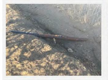
**Photograph 11.** A pipeline under the unnamed dirt road/trail on the subject property is exposed due to erosion. The pipeline is likely associated with a historical water tank.
