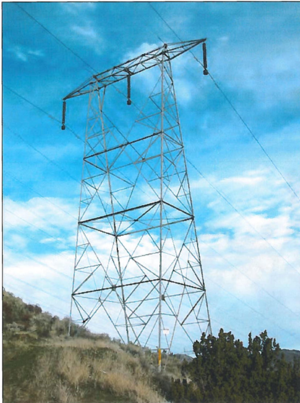
Tower Type #1: Suspension (Standard) Vincent Tower (M18-T1).
