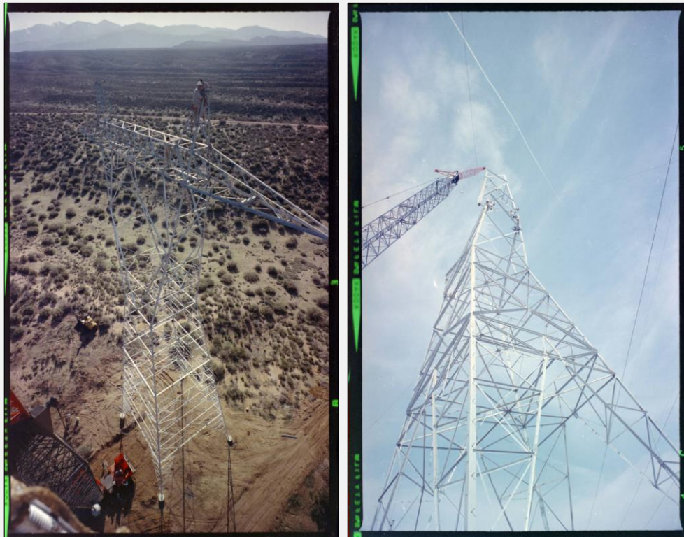
Exhibit 2. Lugo-Vincent 500kV towers under construction, 1968.
