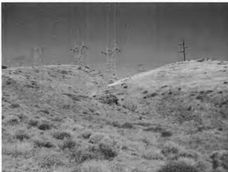
View west of Sagebrush line (right) and Vincent Line (center) in Anaverde Valley in the eastern Sierra Pelona
