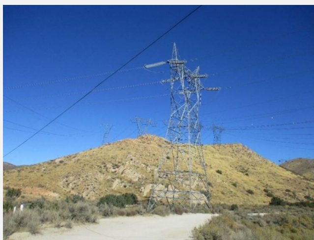
Photograph 1. Tower of the Midway-Vincent No. 1 and No. 2, view looking northeast
