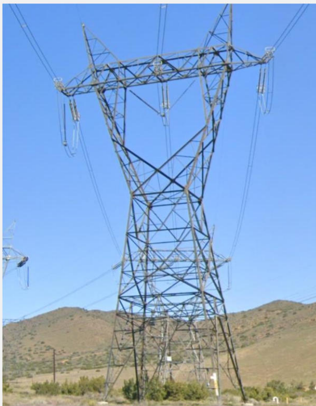
Photograph 2. Tower of the Midway-Vincent No. 1 and No. 2, view looking northeast
