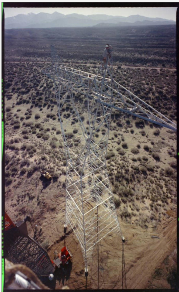
Exhibit 1. Lugo-Vincent 500kV towers under construction, 1968
