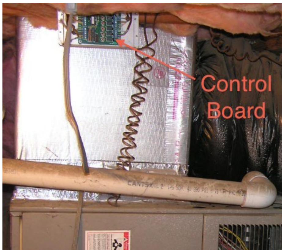
Figure C-6: Photo of a Duct-Mounted Control Board
