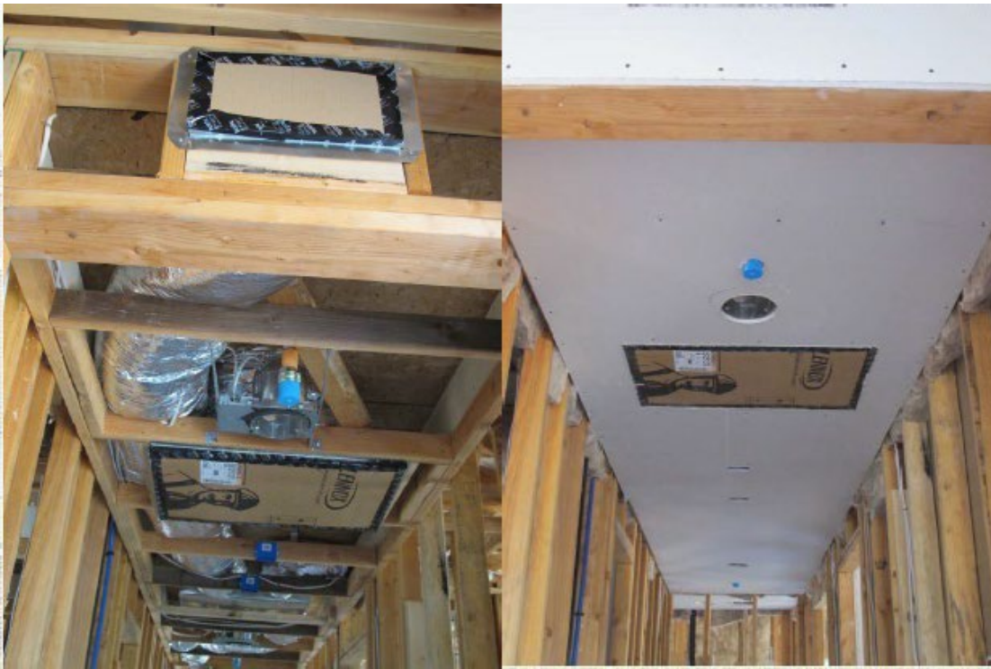
Figure 4-7: Ducts Routed Through a Dropped Ceiling
