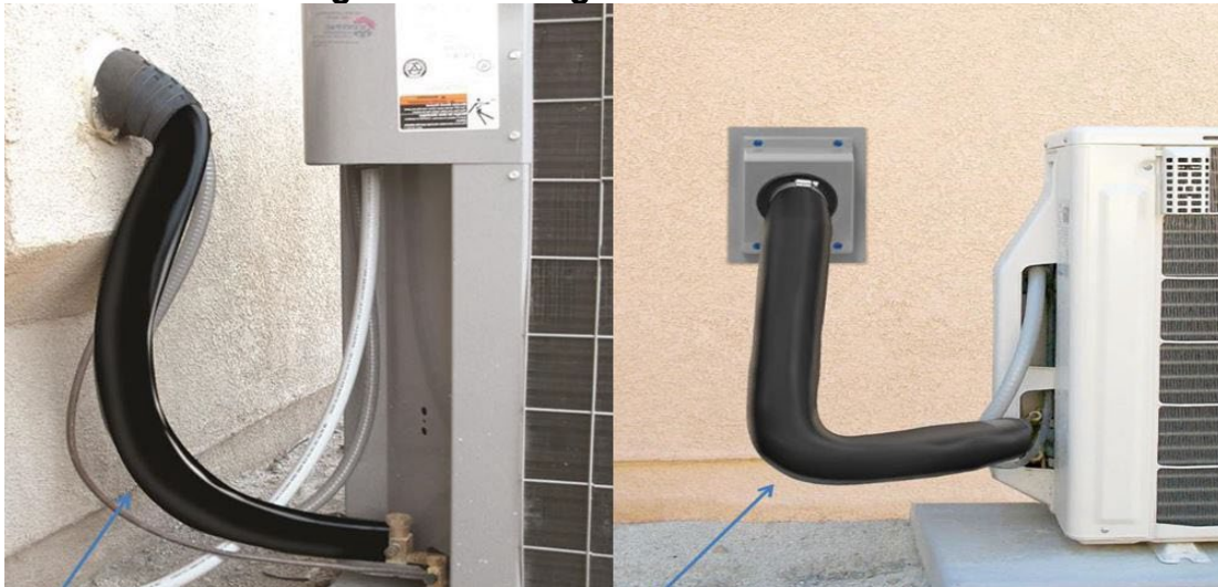
Figure 4-1: Refrigerant Line Insulation
